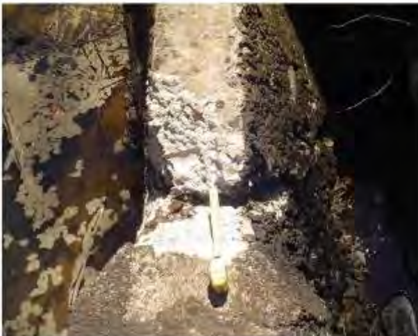
Plate 5 - Crack in the weir wall at Ch 15.5
