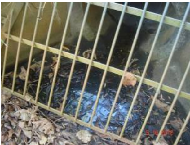
Photo 7 – inlet area at inlet pipe (5/10/12)
