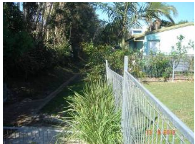
Photo 14 – affect of subsidence on boundary fencing (13/9/12)
