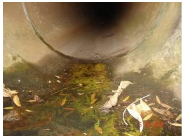
Photo 8 – inlet pipe at inlet area (5/10/12)
