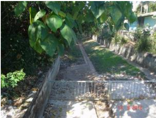
Photo 5- inlet area and v-drain following maintenance and long dry period (13/9/12)
