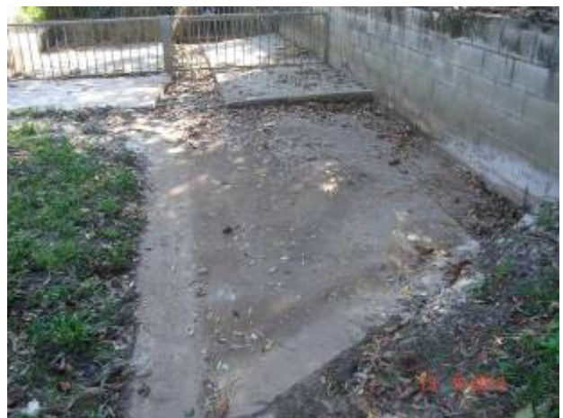
Photo 2 – inlet area following maintenance and long period without rain (13/9/12)
