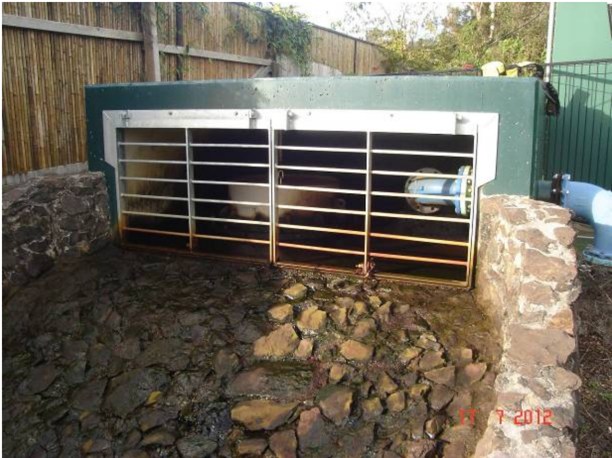
Photo 15 – rock lined drainage chute for flood and sump pump (17/7/12)
