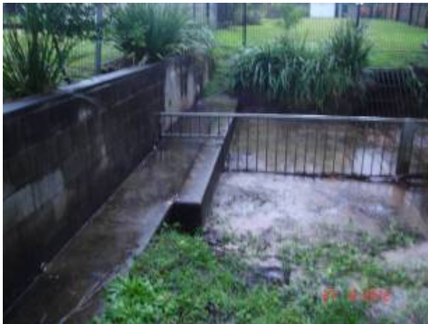
Photo 11 – lower and upper retaining walls near subsidence (27/6/12)
