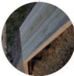
Elements ramping over trunks
