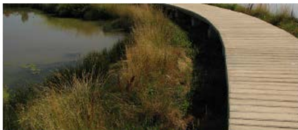
Boardwalks provide access across wetlands
