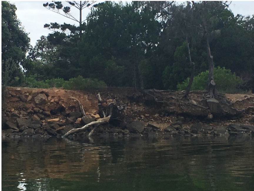
Photo – SI08 failing rock wall
