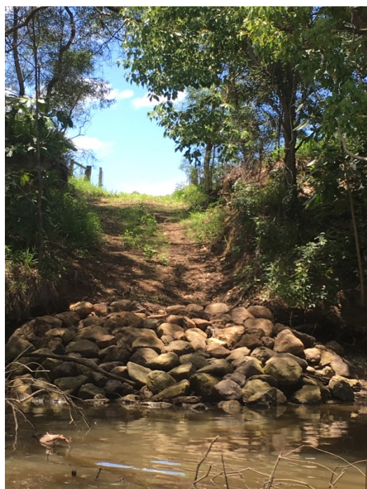
Photos – Site BR06 showing rock ramp revetment/pathway.
