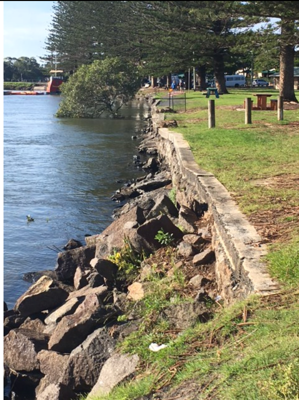
Photo - Si09 failing rock wall
