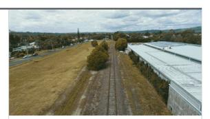
Since rail services were suspended in 2004, there has been little maintenance but also little usage, hence the condition of the track elements remain relatively unchanged, subject only to deterioration from exposure to environmental conditions and vegetation overgrowth.
