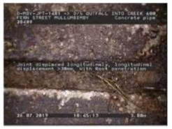
Figure 473 | Displacement, Chg 3.88m
