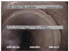
Figure 346 | Displacement, Chg 0.75m
