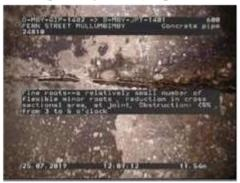
Figure 461 | Root intrusion, Chg 11.54m
