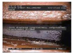
Joint displaced radially radial displacement florance at 8 projects
