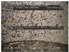
Figure 340 | Cracking, Chg 1.14m
