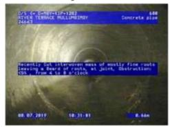
Figure 259 |Root intrusion, Chg0.66m
