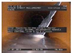
Figure 605 | Pipe section missing, Chg 8.71m
