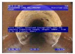
Figure 523 | Patch liner, Chg 72.13m
