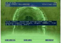
Figure 54 | Infiltration, Chg 14.89m
