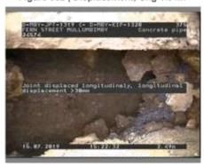
Figure 354 | Displacement, Chg 2.49m
