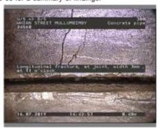
Figure 369 | Cracking, Chg 0.48m
