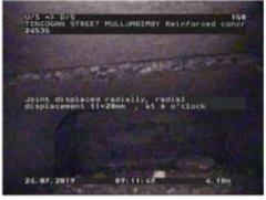
Figure 434 | Displacement, Chg 4.18m
