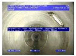
Figure 26 | Lifting eye seal, Chg16.11m
