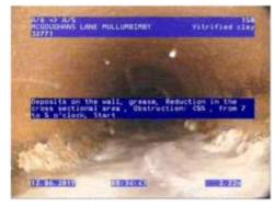
Deposits on the wall, Encrestation above the waterline, Costruction: CSS , from 7 to S o'clock
