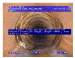
Figure 518 | Patch liner, Chg 52.04m
