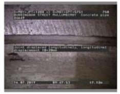
Figure 363 | Displacement, Chg 4.72m
