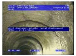
Figure 265 | Displacement, Chg11.73m
