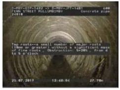
Figure 465 | Root intrusion, Chg 27.70m
