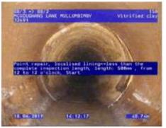
Figure 516 | Patch liner, Chg 48.74m
