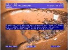
Figure 84 | Radial displacement, Chg 11.18m
