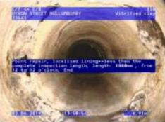
Figure 69 | Patch liner, Chg 6.14m
