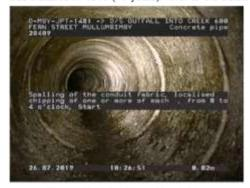
Figure 470 | Spalling, Chg 0.02m
