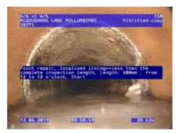
Figure 284 | Patch liner, Chg 28.62m
