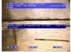
Figure 243 |Reinforcement, Chg31.46m
