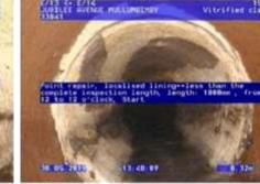
Figure 38 | Liner patch, Chg 45.10m
