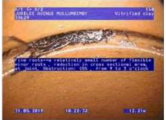
Figure 50 | Root intrusion, Chg 4.59m
