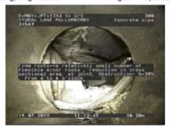
Figure 414 | Root intrusion, Chg 30.20m
