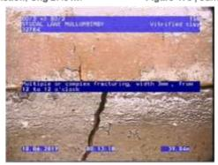
Figure 477 | Cracking, Chg 39.84m
