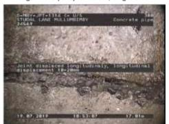
Figure 411 | Displacement, Chg 17.01m
