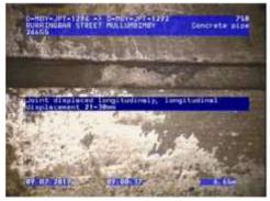
Figure 300 |Displacement, Chg6.65m
