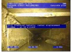
Figure 168 | Displacement, Chg3.32m
