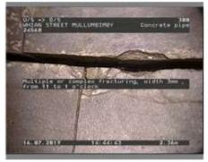
Figure 371 | Cracking, Chg 2.36m
