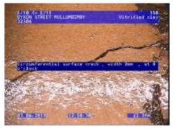
Figure 68 | Cracking, Chg 42.39m
