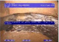
Figure 184 | Cracking, Chg 37.45m
