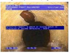
Figure 338 | Patch liner, Chg 27.34m
