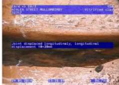
Figure 16 | Cracking, Chg 44.57m
