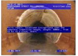
Figure 332 | Patch liner, Chg 6.91m
