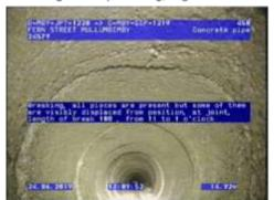
Figure 103 |Crushing, Chg12.38m
