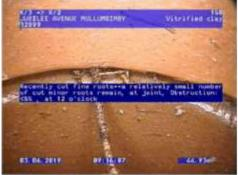
Figure 60 | Root intrusion, Chg 0.04m
