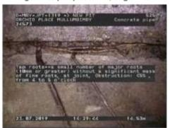
Figure 422 | Root intrusion, Chg 14.53m
