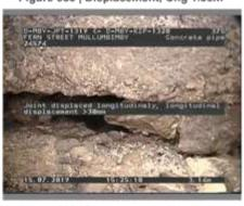
Figure 355 | Displacement, Chg 3.14m
