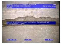
Figure 285 | Displacement, Chg6.47m
