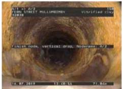
Figure 586 | Patch liner, Chg 70.94m
