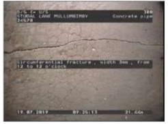
Figure 398 | Cracking, Chg 21.44m
