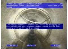
Figure 45 |Lifting eye seal, Chg0.54m
