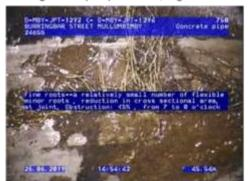
Figure 131 | Infiltration, Chg44.08m
