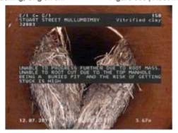
Figure 539 | Root intrusion, Chg 3.67m
