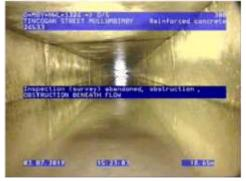
Figure 225 |Displacement, Chg2.40m
