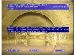
Figure 213 | Displacement, Chg2.38m
