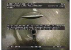
Figure 443 | Displacement, Chg 16.92m
