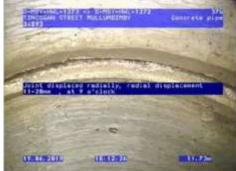
Figure 2 |Pipe breaking, Chg7.14m
