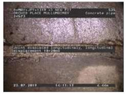
Figure 419 | Displacement, Chg 4.44m
