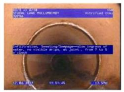
Figure 433 | Infiltration, Chg 13.59m
