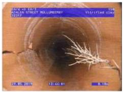
Figure 12 | Cracking, Chg 8.07m
