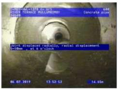
Figure 257 |Root intrusion, Chg12.03m
