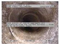
Figure 344 | Aggregate, Chg 0.00m
