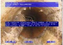
Figure 2 | Liner in poor condition, Chg 0.07m
