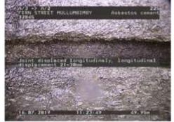
Figure 572 | Displacement, Chg 49.95m
