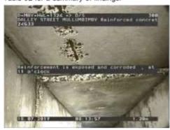
Figure 379 | Reinforcement, Chg 1.20m
