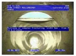
Figure 121 | Defective repair, Chg24.25m
