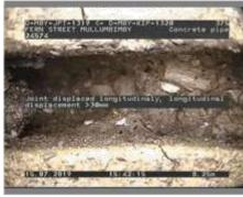
Figure 357 | Displacement, Chg 8.25m
