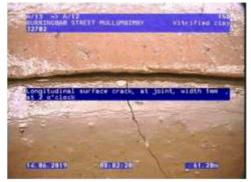
Figure 406 | Cracking, Chg 61.20m
