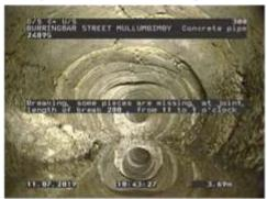
Figure 330 | Deformation, Chg 3.69m
