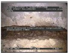
Figure 352 | Displacement, Chg 1.84m
