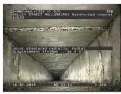
Figure 380 | Displacement, Chg 7.47m
