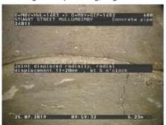
Figure 452 | Displacement, Chg 5.23m
