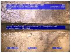
Figure 175 | Displacement, Chg4.39m
