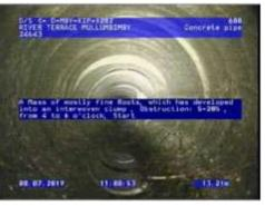
Figure 268 |Root intrusion, Chg13.21m
