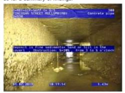
Connection, poor workmanship, cornection appears to be open, dismeter 225mm, width 725mm
