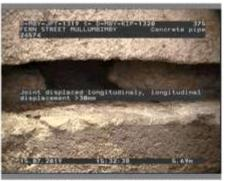
Figure 356 | Displacement, Chg 5.69m
