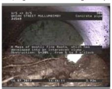
Figure 372 | root intrusion, Chg 3.92m
