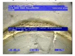
Figure 313 |Displacement, Chg2.92m
