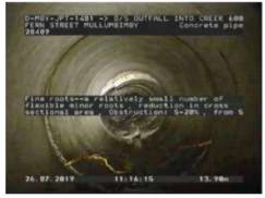
Figure 478 | Root intrusion, Chg 13.90m
