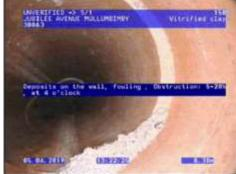
Figure 119 | Circumferential crack, Chg 0.38m
