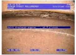
Figure 97 | Cracking/infiltration, Chg 1.71m
