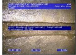
Figure 273 |Cracking, Chg0.60m
