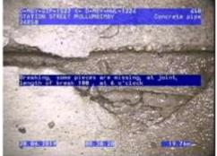
Figure 20 |Infiltration, Chg18.56m
