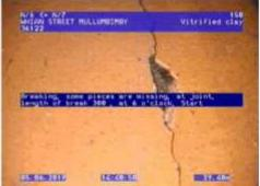
Figure 129 | Cracking, Chg 29.15m
