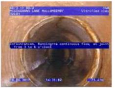
Figure 522 | Infiltration, Chg 71.41m
