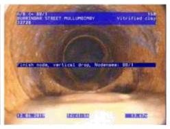
Figure 358 | Radial displacement, Chg 13.53m
