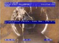
Figure 31 | Cracking and root intrusion Chg 53.40m
