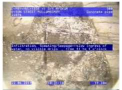
Figure 83 | Cracking, Chg16.82m
