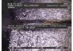
Figure 568 | Displacement, Chg 37.08m
