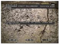
Figure 327 | Cracking, Chg 1.05m
