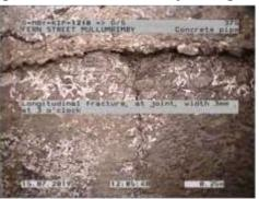
Figure 345 | Cracking, Chg 0.25m
