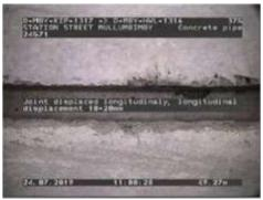
Figure 440 | Displacement, Chg 49.27m
