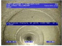
Figure 105 | Cracking, Chg18.08m
