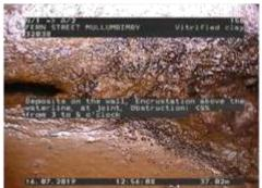
Figure 578 | Infiltration, Chg 26.48m
