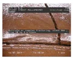
Figure 528 | Cracking, Chg 1.66m
