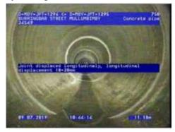
Figure 304 | Displacement, Chg1.37m
