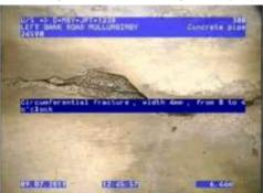
Figure 315 |Cracking, Chg6.44m
