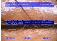
Figure 101 | Cracking, Chg 0.32m
