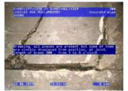
Figure 89 | Cracking, Chg5.57m
