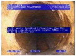
Figure 521 | Patch liner, Chg 65.17m
