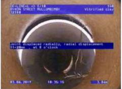
Figure 62 | Root intrusion, Chg 1.17m
