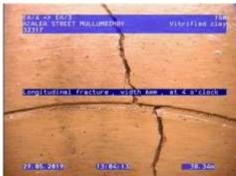
Figure 14 | Cracking, Chg 25.46m
