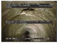
Figure 460 | Cracking, Chg 4.62m
