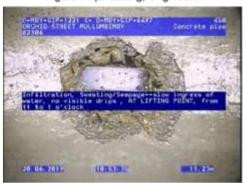
Figure 32 | Lifting eye seal, Chg8.79m
