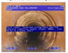
Figure 520 | Patch liner, Chg 63.86m
