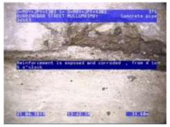
Figure 55 |Reinforcement, Chg11.87m
