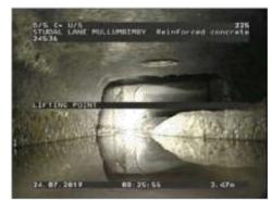
Figure 428 | Displacement, Chg 3.01m
