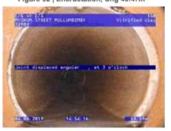
Figure 93 | Long Displacement, Chg 57.73m
