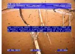
Figure 189 | Root intrusion, Chg 15.97m
