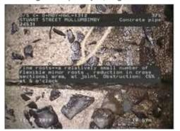
Figure 334 | Root intrusion, Chg 3.29m
