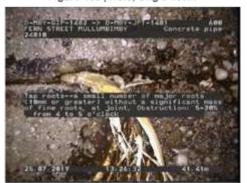
Figure 468 | Root intrusion, Chg 41.41m
