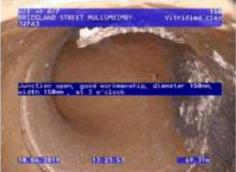
Figure 263 | Cracking, Chg 55.03m
