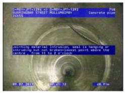
Figure 302 |Displacement, Chg23.76m
