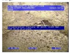
Figure 143 (Cracking, Chg0.11m
