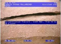
Figure 117 | Radial displacement, Chg 52.23m
