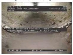
Figure 395 | Displacement, Chg 12.76m
