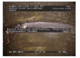
Figure 427 | Displacement, Chg 29.38m
