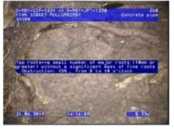
Figure 63 |Broken pipe, Chg8.33m
