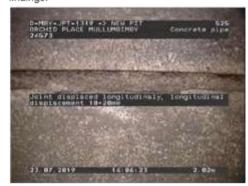
Figure 418 | Displacement, Chg 2.02m
