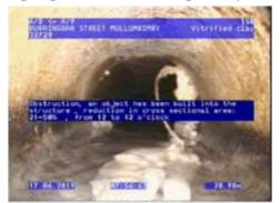
Figure 376 | Defective patch liner, Chg 49.51m
