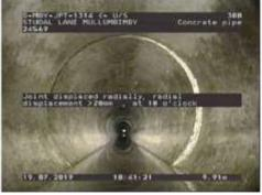
Figure 409 | Displacement, Chg 9.91m
