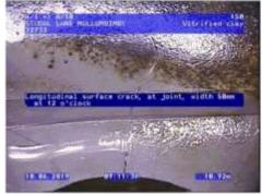
Figure 231 | Pipe replacement, Chg 10.92m
