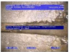
Figure 287 | Displacement, Chg10.83m
