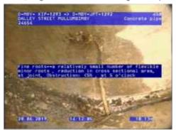
Figure 165 | Root intrusion, Chg10.13m
