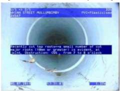
Figure 251 | Root intrusion, Chg1.37m
