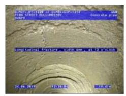
Figure 106 | Cracking, Chg19.41m
