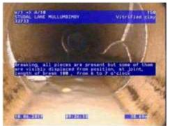
Figure 235 | Cracking, Chg 34.21m
