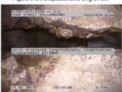
Figure 348 | Displacement, Chg 3.93m
