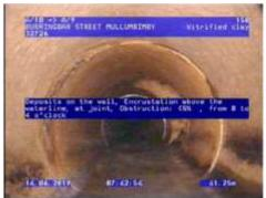
Figure 368 | Infiltration, Chg 28.07m
