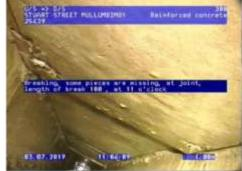
Figure 215 |Displacement, Chg1.00m
