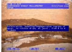
Figure 366 | Infiltration, Chg 25.27m
