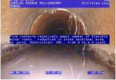
Figure 227 | Root intrusion, Chg 48.16m
