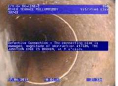
Figure 423 | Defect, Chg 21.16m
