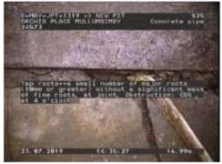
Figure 424 | Root intrusion, Chg 16.99m
