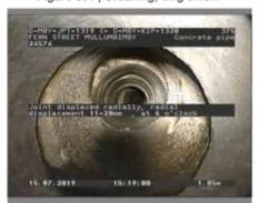
Figure 353 | Displacement, Chg 1.85m
