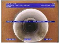
CONNECTION, Good workmanship, Connection agreers to be open, Glameter 150ms, width 100ms, at 12 o'clock
