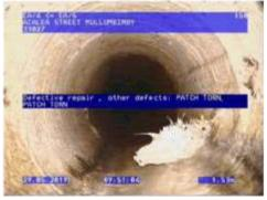
Figure 5 | Torn liner, Chg 1.53m
