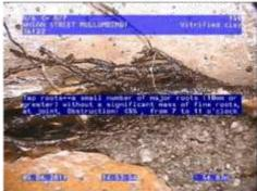
Figure 131 | Cracking / roots, Chg 29.70m
