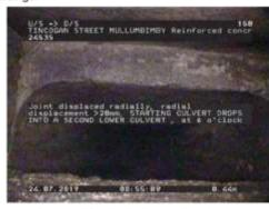
Figure 432 | Vertical step, Chg 0.44m
