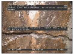
Figure 404 | Cracking, Chg 3.79m
