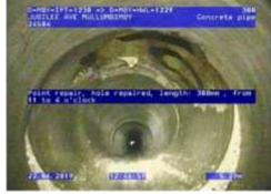
Figure 87 |Displacement, Chg5.02m
