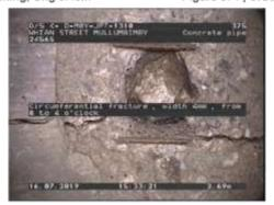
Figure 375 | Cracking, Chg 2.69m
