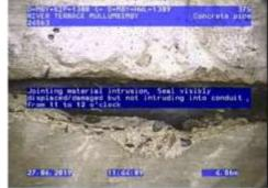
Figure 133 |Lifting eye seal, Chg0.94m
