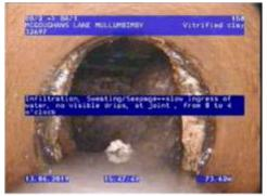
Figure 399 | Infiltration/encrustation, Chg 73.62m
