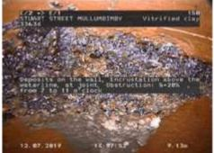
Figure 544 | Displacement, Chg 8.17m
