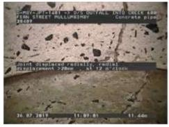
Figure 476 | Displacement, Chg 11.44m
