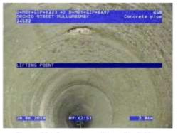
Figure 29 |Lifting eye seal, Chg2.05m
