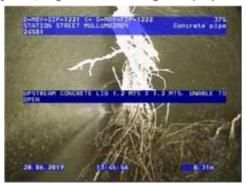
Figure 37 | Significant root intrusion, Chg 8.31m
