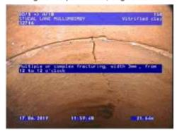
Figure 435 | Cracking, Chg 21.66m
