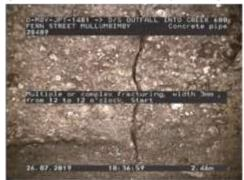
Figure 471 | Cracking, Chg 2.46m
