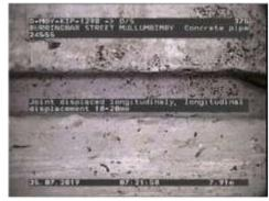
Figure 445 | Displacement, Chg 2.88m
