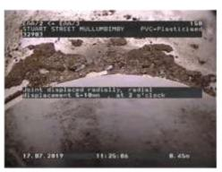
Figure 600 | Displacement, Chg 0.45m
