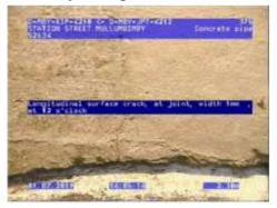
Figure 186 |Typical condition, Chg0.50m
