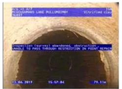
Figure 276 | Patch liner, Chg 74.82m
