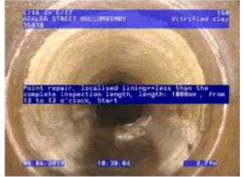
Figure 218 | Patch liner, Chg 53.18m
