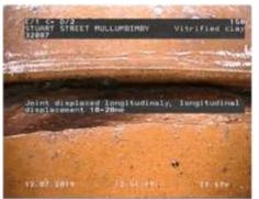
Figure 532 | Displacement, Chg 19.69m
