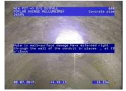
Figure 294 | Displacement, Chg15.28m
