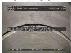
Figure 396 | Displacement, Chg 15.15m
