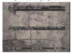
Carcomferential fracture width 2mm, from to 6 of cook
