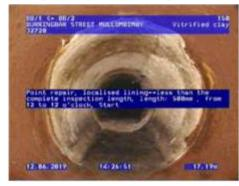
Point repair. Iscalined lining rises than the complete inspection length; tength; \$90mm, from 12 to 12 o'clock, Start
