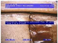
Figure 385 | Infiltration, Chg 20.21m
