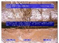
Figure 103 | Root intrusion, Chg 49.84m
