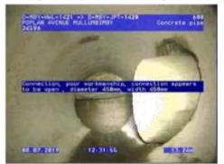
Figure 281 | Displacement, Chg9.95m
