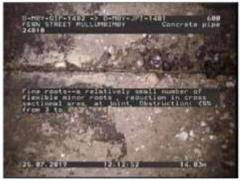
Figure 462 | Root intrusion, Chg 14.03m
