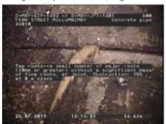
Figure 463 | Root intrusion, Chg 14.61m
