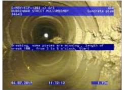
Figure 233 |Cracking, Chg1.73m
