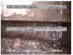
Figure 349 | Displacement, Chg 5.78m
