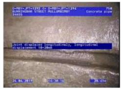
Figure 129 | Infiltration, Chg9.91m
