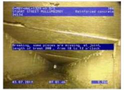
Figure 205 | Cracking, Chg7.37m
