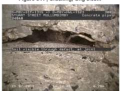
Figure 342 | Displacement, Chg 4.15m
