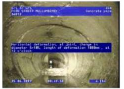
Figure 113 |Displacement, Chg3.69m
