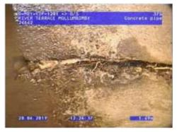
Figure 161 | Cracking, Chg1.13m
