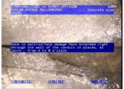
Figure 279 |Displacement, Chg4.97m
