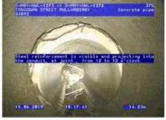
Figure 4 | Exposed reinforcement, Chg14.23m
