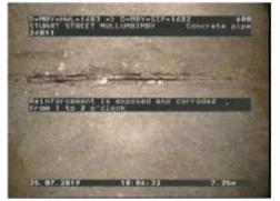
Figure 453 | Reinforcement, Chg 7.25m
