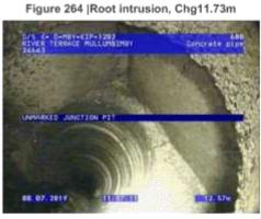
Figure 266 |Unmarked MH, Chg12.57m
