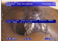
Figure 340 | Root intrusion, Chg 0.85m
