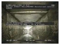
Figure 381 | Displacement, Chg 28.57m
