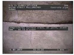
Figure 373 | Cracking, Chg 0.45m
