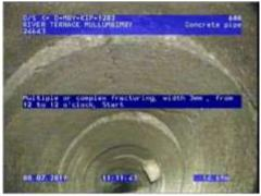
Figure 269 | Cracking, Chg14.69m
