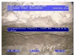
Figure 54 (Cracking, Chg63.81m
