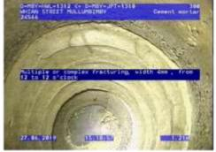
Figure 145 | Displacement, Chg1.11m
