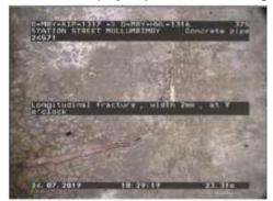
Figure 436 | Cracking, Chg 23.31m
