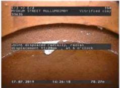
Figure 609 | Displacement, Chg 78.27m
