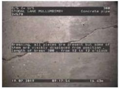
Figure 397 | Cracking, Chg 16.43m
