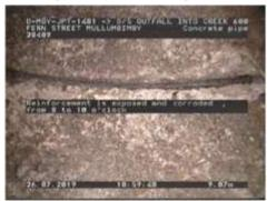
Figure 474 | Reinforcement, Chg 9.07m
