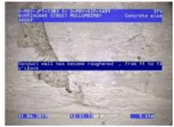
Figure 57 |Cracking, Chg0.83m
