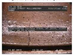
Figure 529 | Cracking, Chg 8.60m
