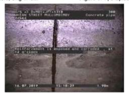
Figure 375 | Reinforcement, Chg 1.98m
