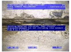
Figure 135 |Lifting eye seal, Chg5.91m
