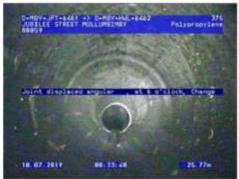
Figure 316 | Displacement, Chg25.77m
