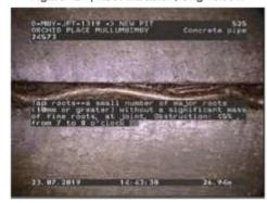
Figure 426 | Root intrusion, Chg 26.94m
