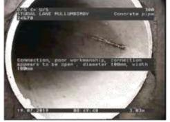
Figure 389 | Cracking, Chg 1.42m
