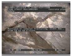
Figure 351 | Cracking, Chg 0.16m
