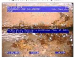
Figure 325 | Infiltration, Chg 13.44m
