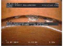
Figure 542 | Displacement, Chg 1.26m
