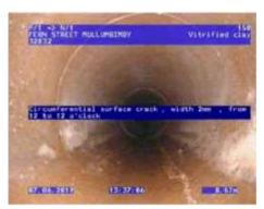
Figure 207 | Cracking, Chg 0.67m
