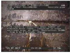
Figure 467 | Root intrusion, Chg 37.70m
