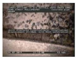
Figure 477 | Displacement, Chg 12.34m
