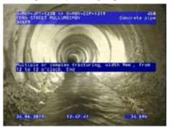
Figure 110 | Cracking, Chg34.69m
