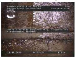
Figure 420 | Displacement, Chg 6.91m
