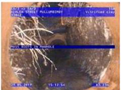
Figure 20 | Cracking and root intrusion, Chg 37.30m
