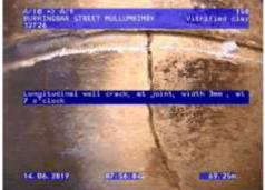
Figure 372 | Cracking, Chg 55.96m
