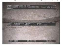
Figure 447 | Displacement, Chg 15.41m
