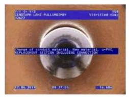
Connection, good workmanship, connection appears to be open, disseler 154mm, width 154mm, at 3 crieck
