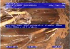
Figure 193 | Root intrusion, Chg 49.51m
