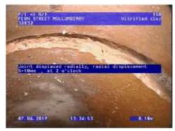
Figure 206 | Radial displacement, Chg 0.10m
