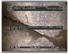
Figure 359 | Cracking, Chg 13.26m
