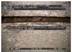
Figure 469 | Displacement, Chg 45.16m
