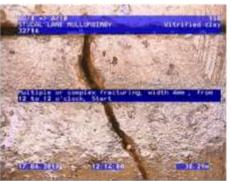
Figure 438 | Cracking, Chg 38.29m
