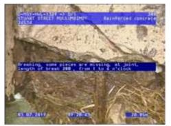
Figure 209 |Cracking, Chg20.05m
