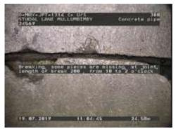
Figure 412 | Cracking, Chg 18.30m
