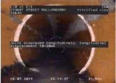
Figure 546 | Displacement, Chg 10.11m
