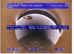
Figure 402 | Infiltration, Chg 24.24m
