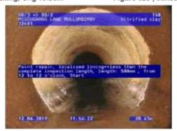
Figure 329 | Patch liner, Chg 20.43m
