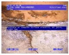
Figure 436 | Cracking, Chg 25.71m
