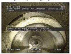
Figure 328 | Displacement, Chg 2.09m
