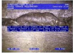
Figure 255 |Root intrusion, Chg2.35m
