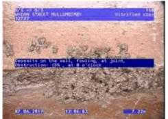
General Du the wall, Encrustation shows the saterline, at joint, Obstruction; CW: from 7 to 5 o'clock
