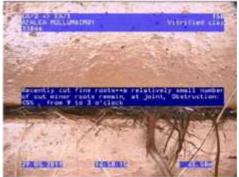
Figure 24 | Cracking and root intrusion, Chg 18.30m
