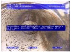
Figure 486 | Displacement, Chg 54.36m
