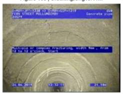
Figure 108 | Cracking, Chg21.18m
