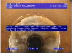
Figure 58 | Patch liner, Chg 35.34m
