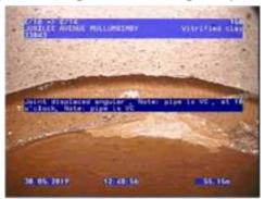
Figure 35 | Angular Displacement, Chg 55.15m
