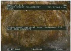
Figure 594 | Displacement, Chg 13.65m
