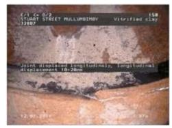
Figure 527 | Displacement, Chg 0.87m
