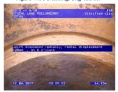
Figure 441 | Infiltration, Chg 55.62m
