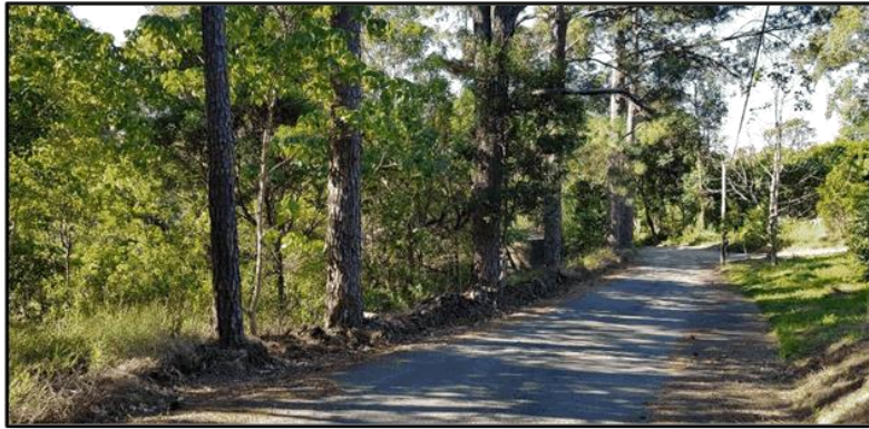
Photo 1 - Sealed road having a 4m unobstructed width in the majority of areas.
