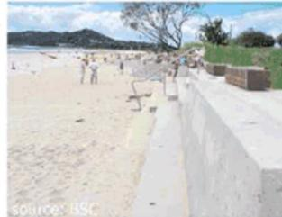
Construction of stepped concrete seawall in front of Apex Park. Steps and formal beach access for disabled and vehicles (e.g. lifeguards).
