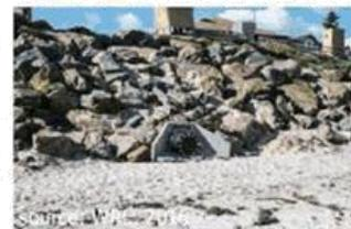
Increase sand bypassing around the structure from east to west via small-scale pumping system. Sand pumping infrastructure built-in to structure.
