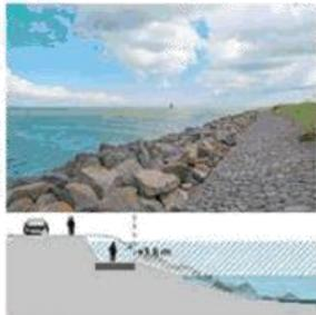
Construction of berm rock revetment with surfaced pathway in front of car park at existing structure alignment. Pathway at level closer to water edge and will be closed during storms. Steps and formal beach access for disabled and vehicles (e.g. lifeguards).
