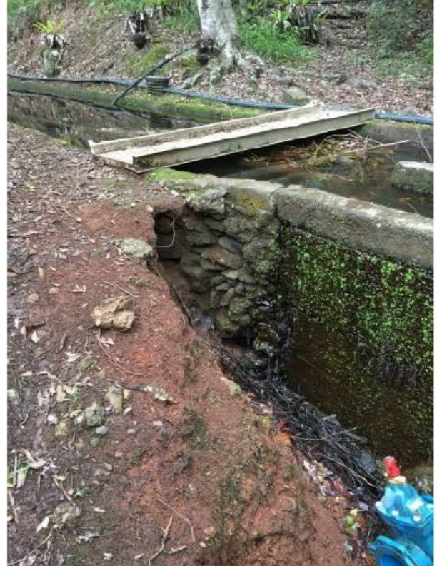
2. Scouring has removed buttressing.
