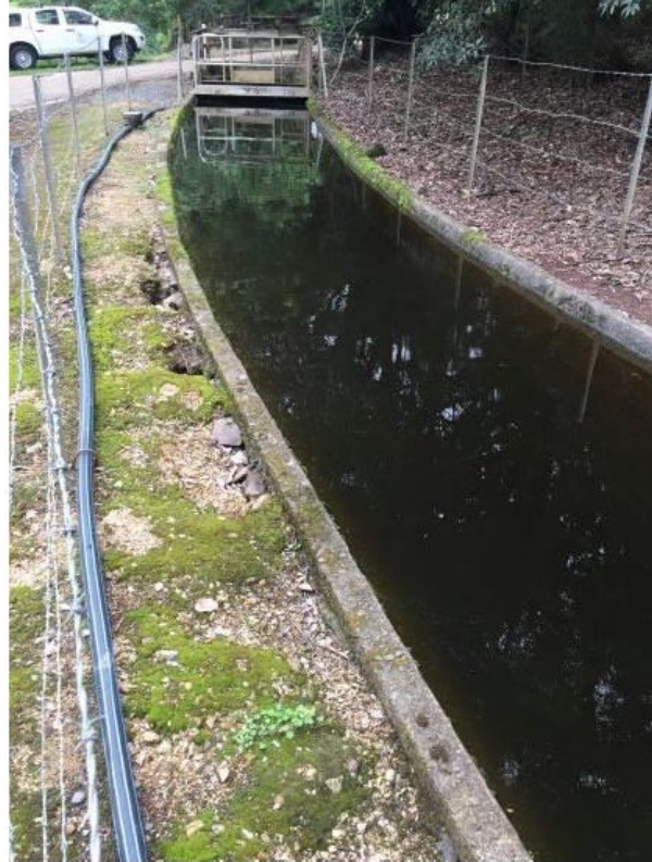
6. Sinkhole formation behind channel wall.
