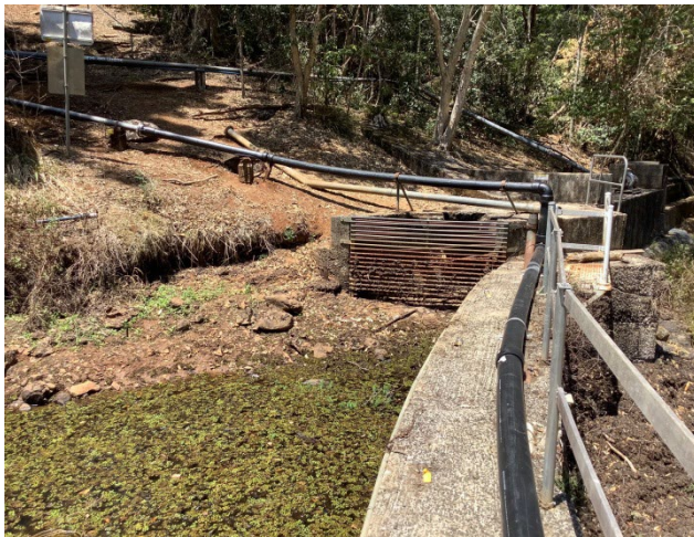
1. Channel inlet (exposed at low weir level)
