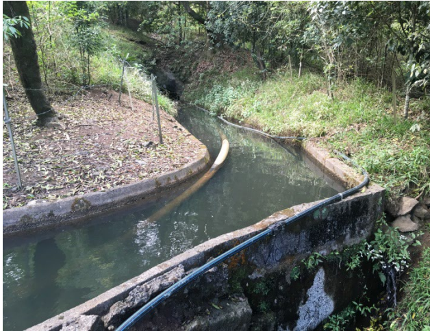
3. Water in channel and leakage from bend
