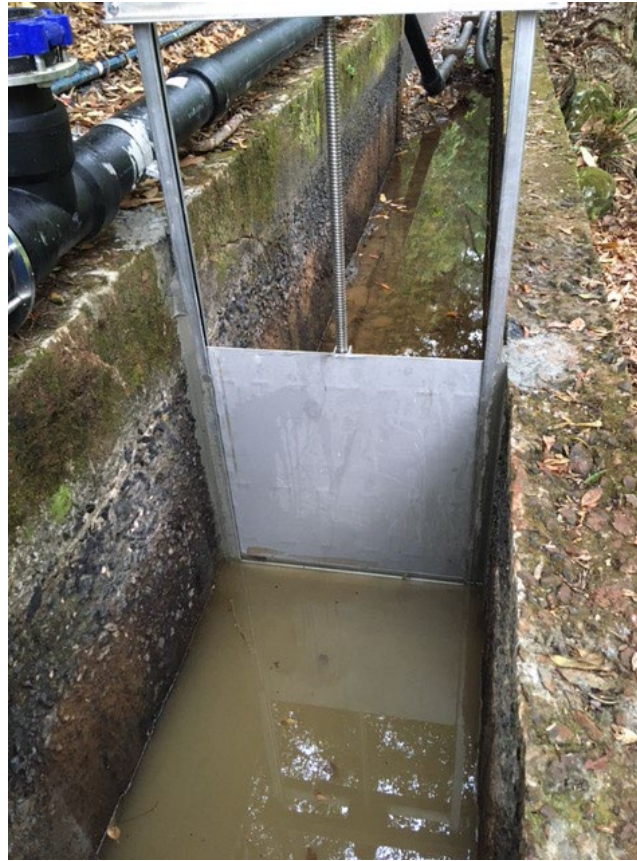
2. New penstock and realigned pump pipework
