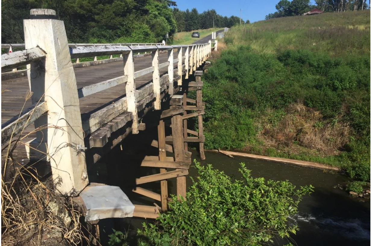
Booyong Bridge (Wilsons River)
