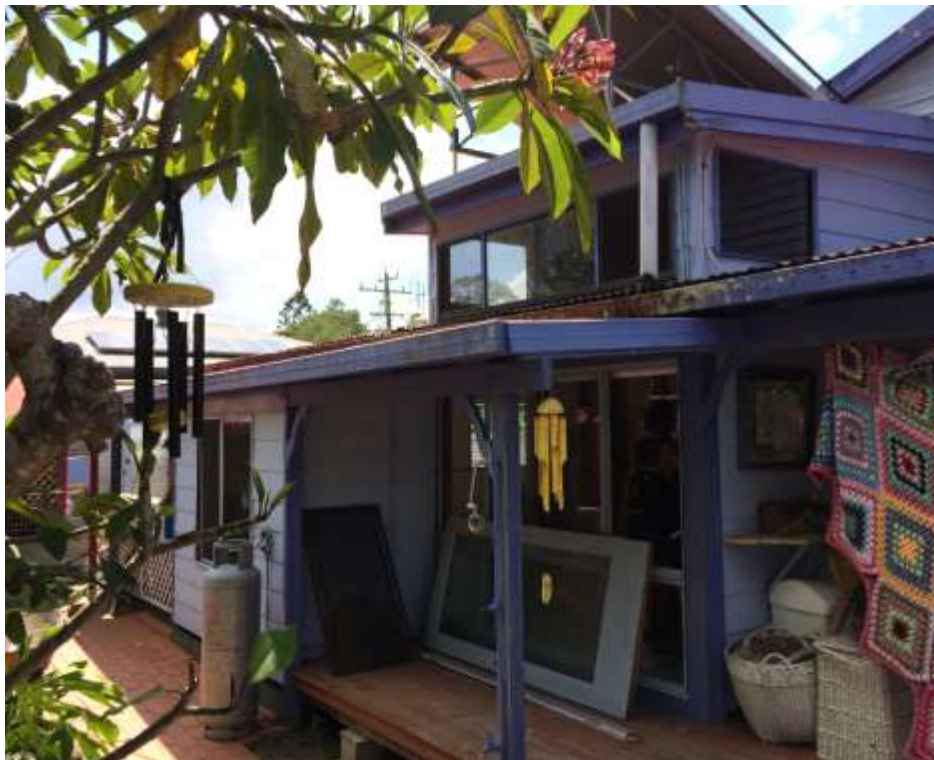
Figure 3: Rear Elevation of existing dwelling
