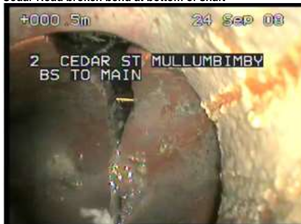
Photograph 10 Cedar Road broken bend at bottom of shaft
