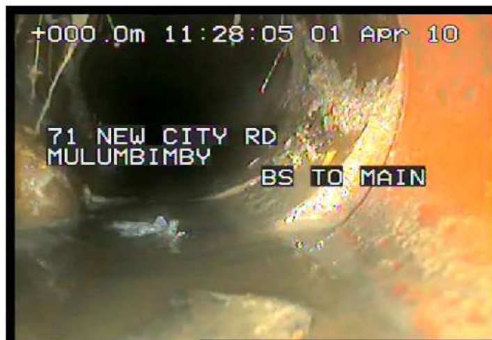
10 Photograph 7 New City Road crack where BS Connects to Main
