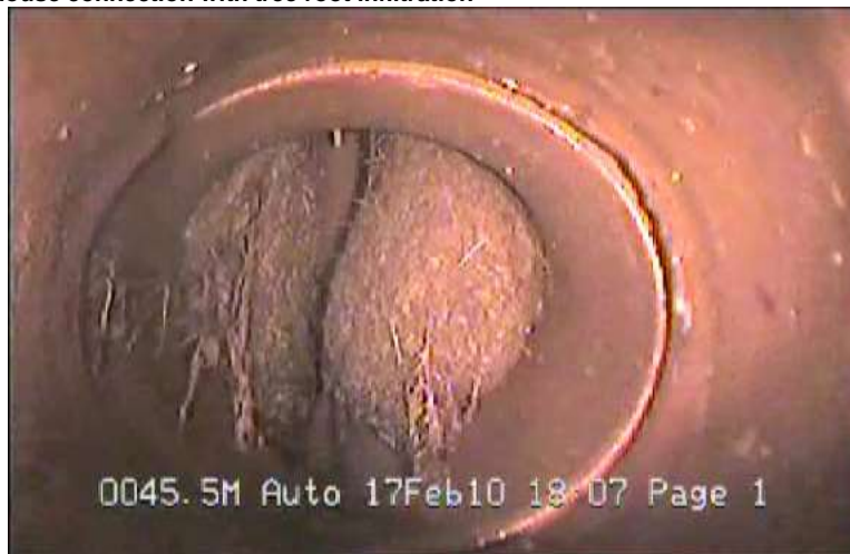
Photograph 8 150mm house connection with tree root infiltration
