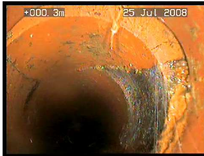
5 Photograph 6 AP14 to AP13-Dislodged joint + Infiltration & tree roots in a 150mm house connection
