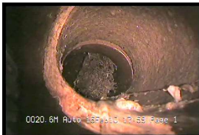
10 Photograph 7 New City Road crack where BS Connects to Main
