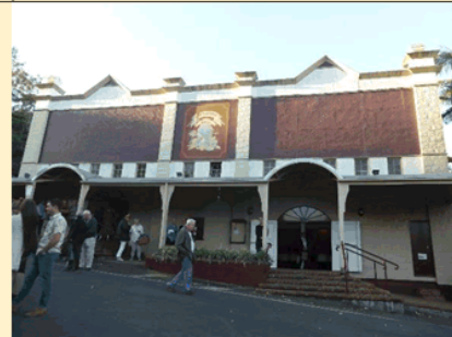
Bangalow A & I Hall. A late Victorian building with pressed metal clad walls.
