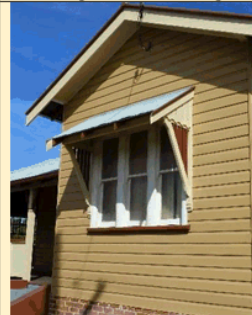
A traditional paint scheme for a timber dwelling based on original paint scrapes.
