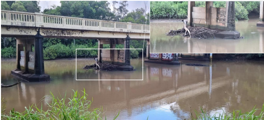
Figure 2.5.1 Debris Accumulation under Federation Bridge (Local Community Member, 2022)
