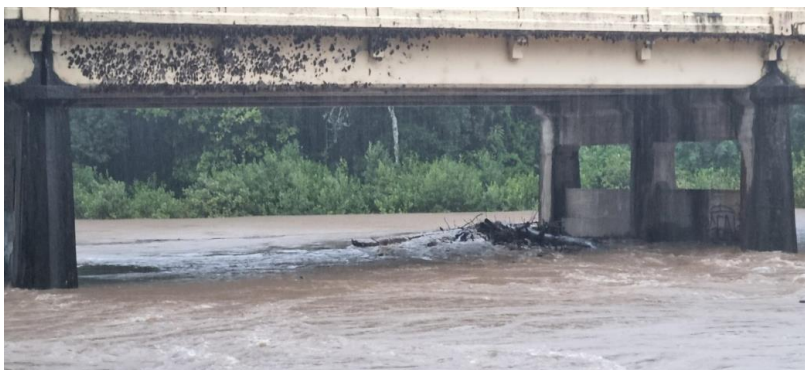
Figure 2.5.2 Debris Accumulation under Federation Bridge during 2022 Flood Event (Local Community Member, 2022)
