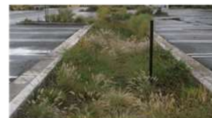
Infiltration beds are effective for flood mitigation.
