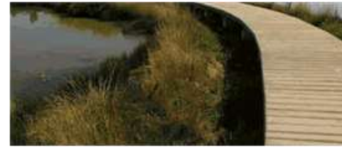
Boardwalks provide access across wetlands
