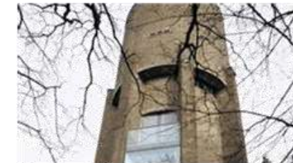
Water Tower adaptive reuse.
