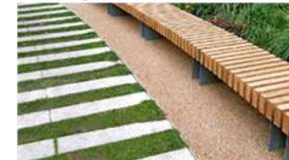
Break down hard surfaces with soft to improve WSUD properties and biodiversity.
