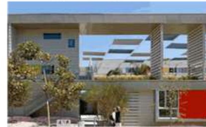
Air Circulation to maintain comfort levels.
