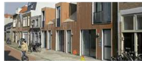
Residential living within the town centre
