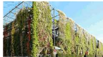
A plant covered Multi-Storey Car 'PARK' facility.
