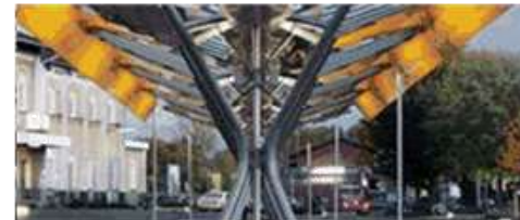
Bus interchange located on the western edge of the railway line
