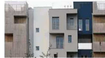
Roof articulation varies street frontages.
