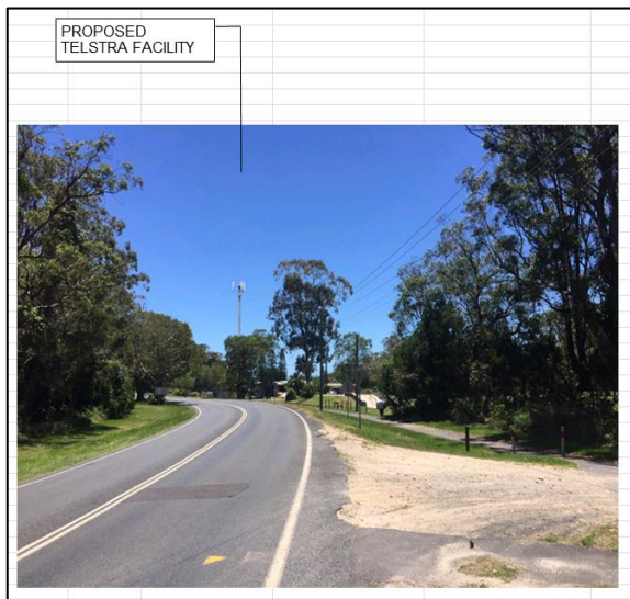
View north along Old Pacific Highway of original proposed location
