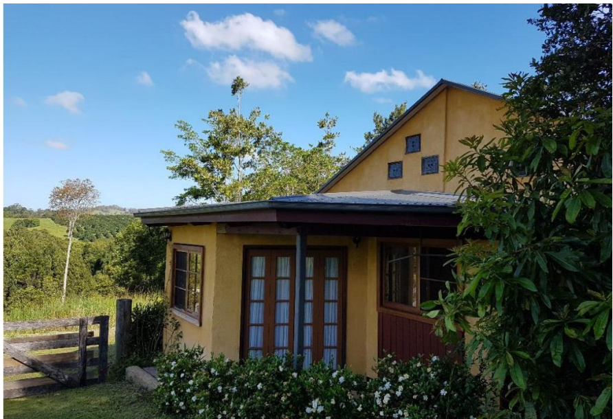
Existing shed structure
