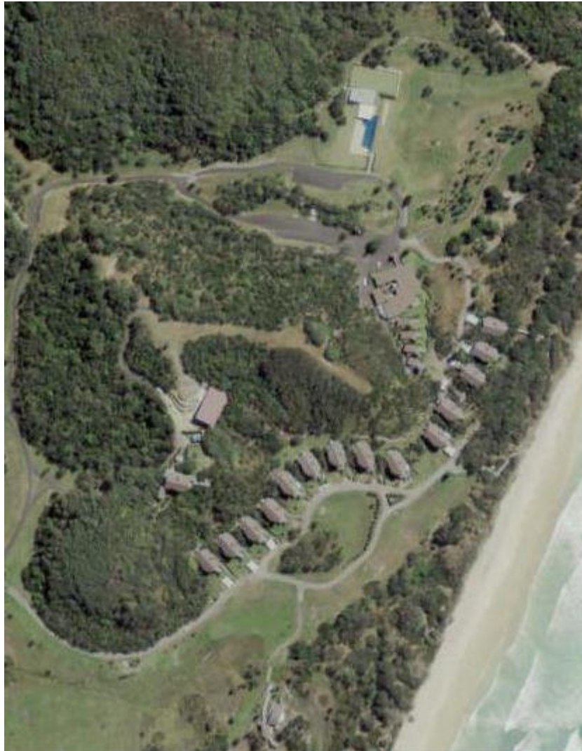
10 Subject site (in part) showing existing structures
