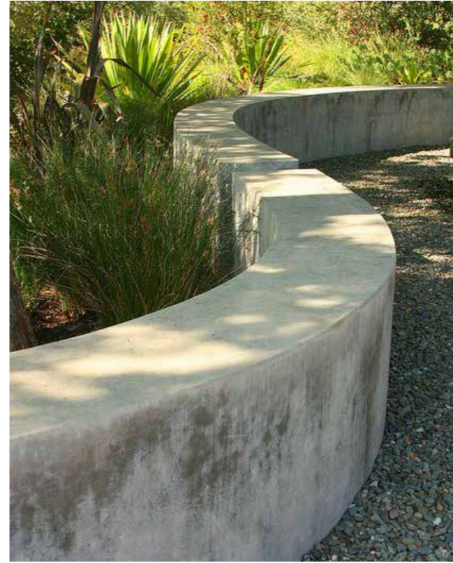
Example of concrete seating wall- play area amenity and barrier
