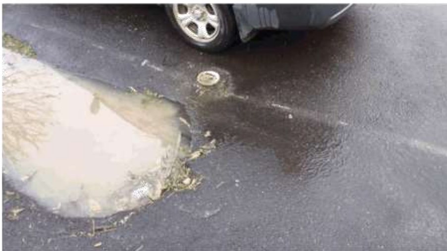
Plate 3 Inspection and observation pit located adjacent to flooded stormwater swale
