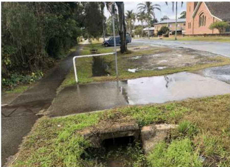
Plate 5 Poor conveyance and lack of maintenance in surface stormwater infrastructure
