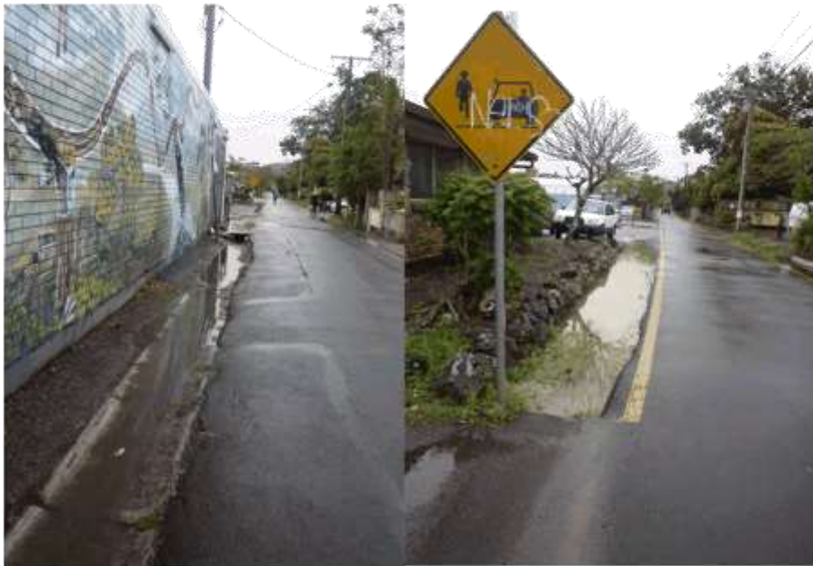
Plate 1 and 2 Poor stormwater conveyance in laneways
