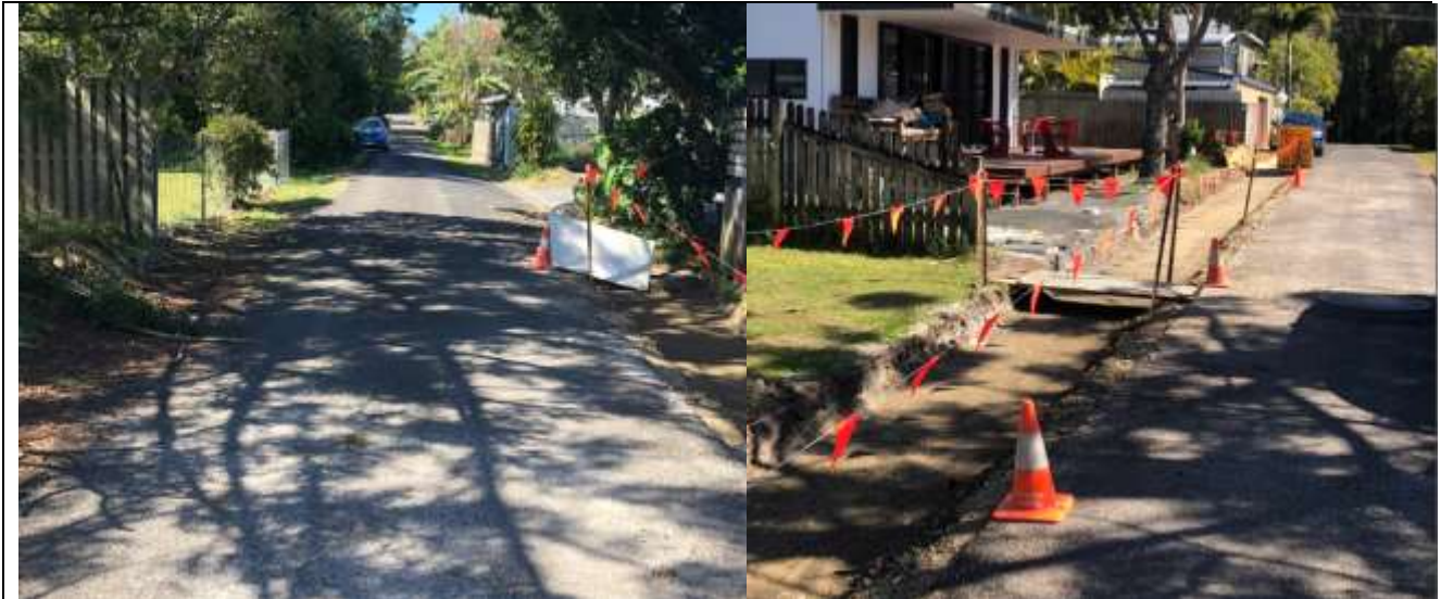
Photo – 7 Galleon Lane – looking east
