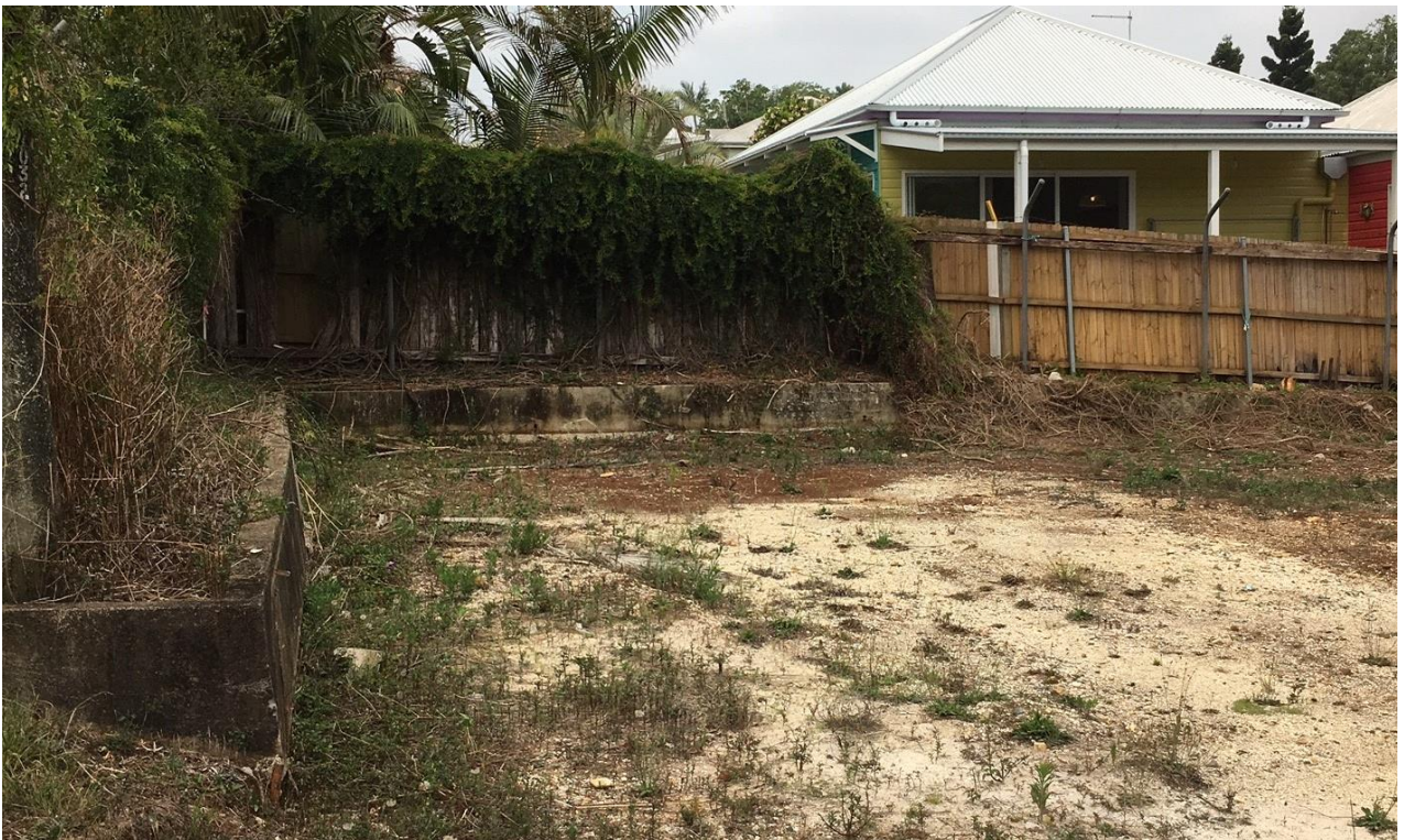
5 Plate 4 – Retaining walls within property
