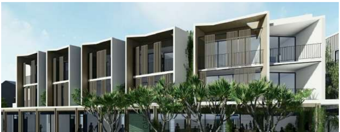
Parapets – Jonson Street frontage
