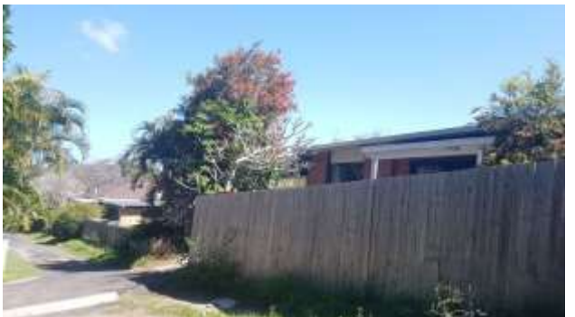
Existing dwellings No. 137 and No. 139 Jonson Street from Ruskin Lane
