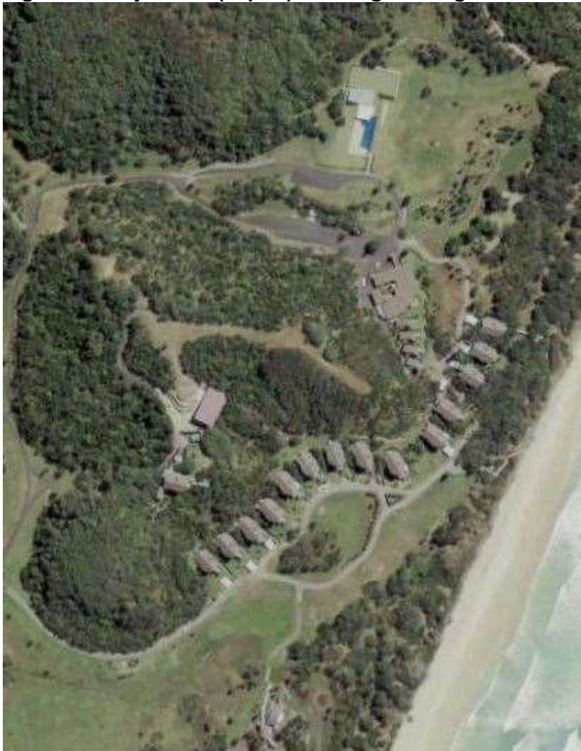
Figure 1: Subject site (in part) showing existing structures
