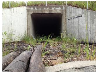
Plate 9. Example of koala floppy top fencing (& refuge pole) to prevent road incursions and to direct fauna to a box culvert underpass (left). Box culvert under the Pacific Highway at Glenugie used on several occasions by koalas (right).
