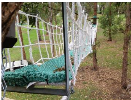
Plate 10. Above road crossing structures targeting koalas – '3-sided' rope bridge on grounds at Southern Cross University (left) and a metal gantry with leaning timber poles over Mt Cotton Road, southeast QLD (right; source: Dexter et al. 2016). Monitoring at both sites did not detect use by koalas.
