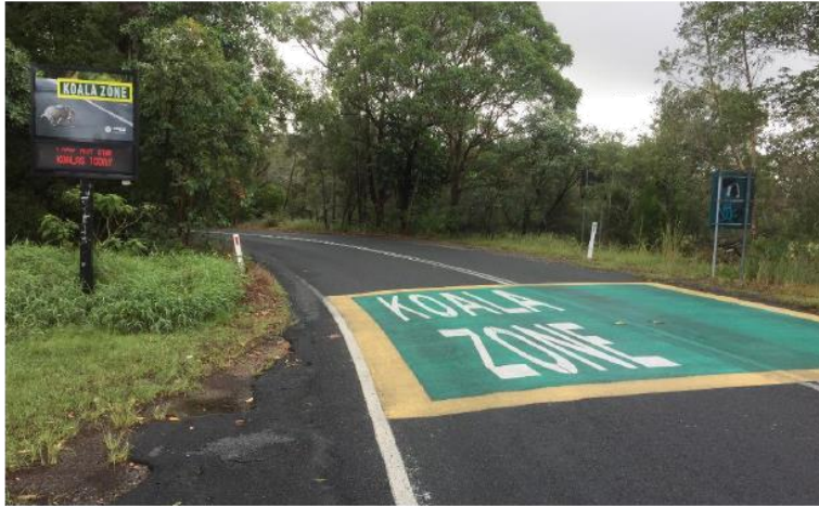
Plate 8. 'Koala Zone' pavement marking (left) and associated VMS sign (right) on Clothiers Creek Road, Tweed LGA.
