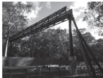
Plate 10. Above road crossing structures targeting koalas – '3-sided' rope bridge on grounds at Southern Cross University (left) and a metal gantry with leaning timber poles over Mt Cotton Road, southeast QLD (right; source: Dexter et al. 2016). Monitoring at both sites did not detect use by koalas.
