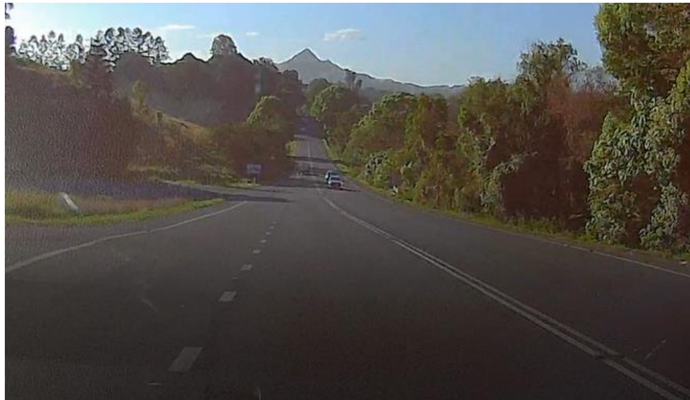
Photo 3: McAuleys Lane/Mullumbimby Road Intersection (looking north along Mullumbimby Road)
