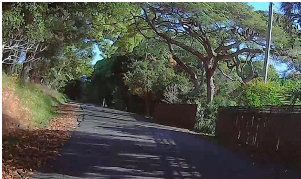
Photo 11: Concealed driveway – driveway through fence at shoulder edge
