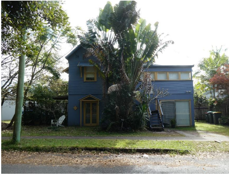
42 The Terrace. A traditional weatherboard dwelling with projecting gable which may have been raised.
