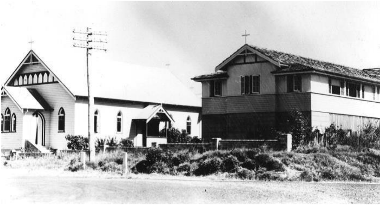
Figure 23 Catholic Church Lady of Lourdes 1936 and adjoining Nuns House 1950 (since demolished)
