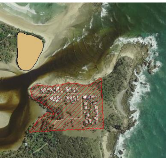
Figure 27 Sandon Village Heritage Conservation Area
