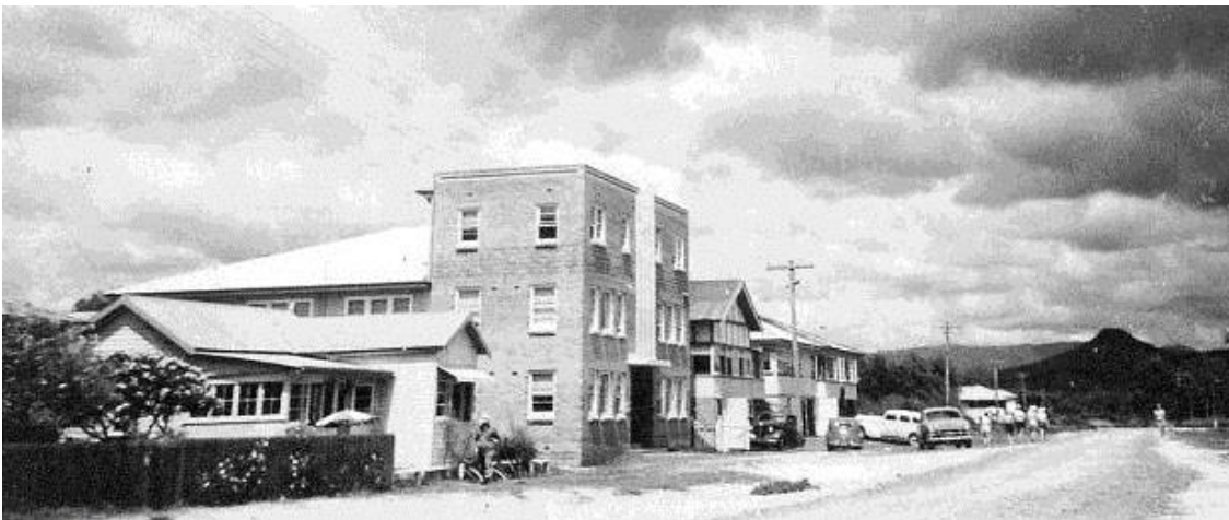
Figure 22 Broadview Flats and adjoining highset houses 1955.
