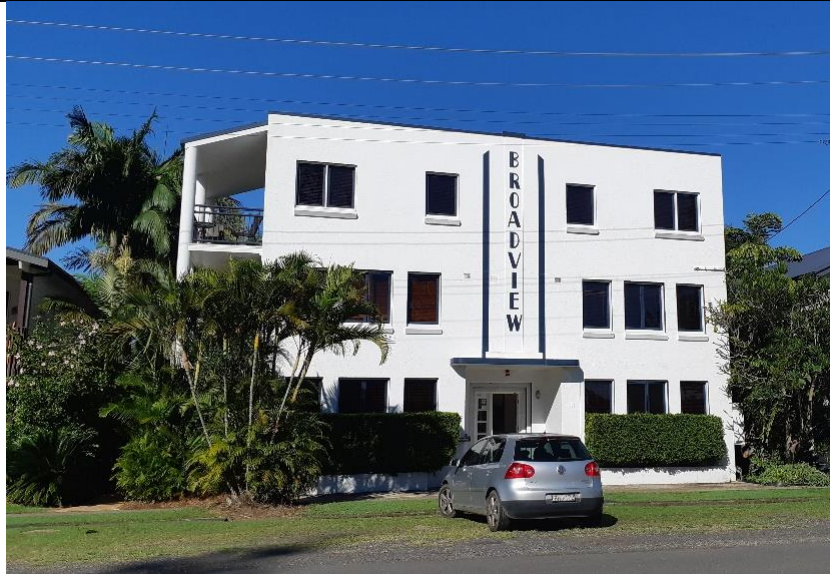
3 "Broadview" flats 12 Fawcett Street
