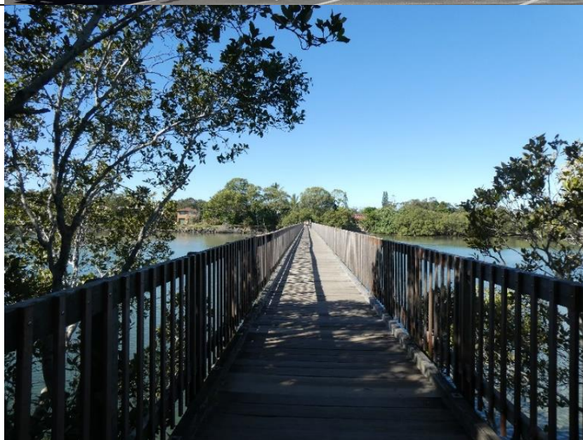
8 Footbridge From The Terrace to South Beach Lane
