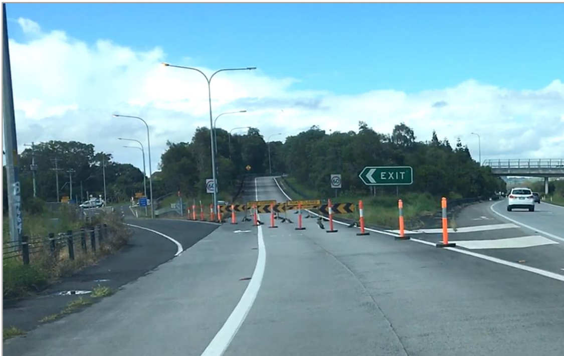
Figure 1 - Southbound off-ramp – Bluesfest 2019, Source: GAA, 18/04/2019
