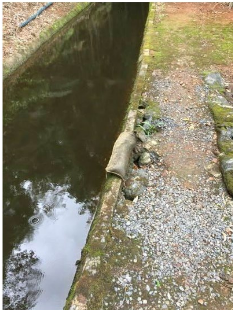
5. Localised slip/subsidence resulting in movement of channel wall.
