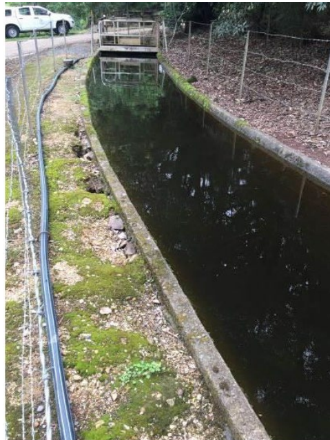
6. Sinkhole formation behind channel wall.
