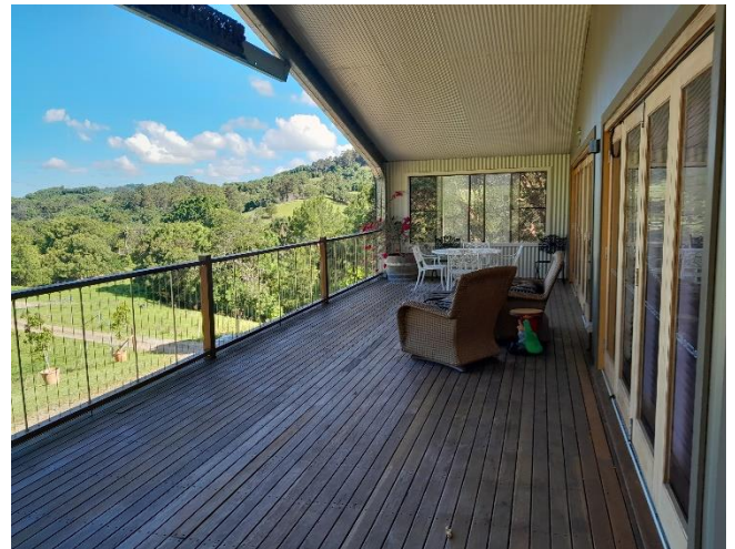
Photo 14 – Building exterior – first floor - balcony
