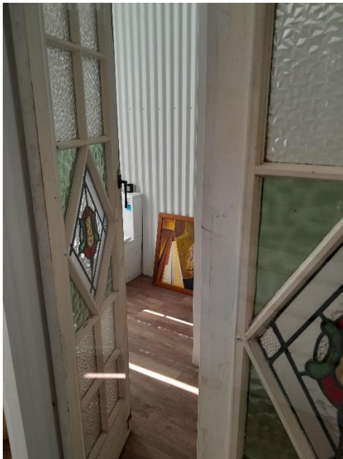
Photo 9 – Building interior – ground floor - bathroom
