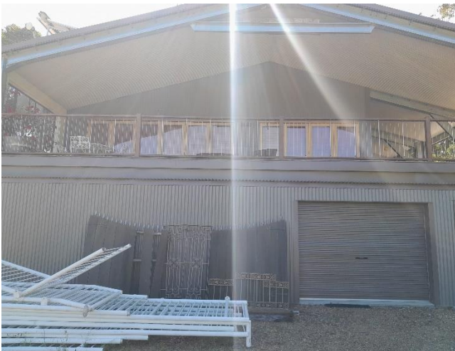
Photo 3 – Building exterior – east facade
