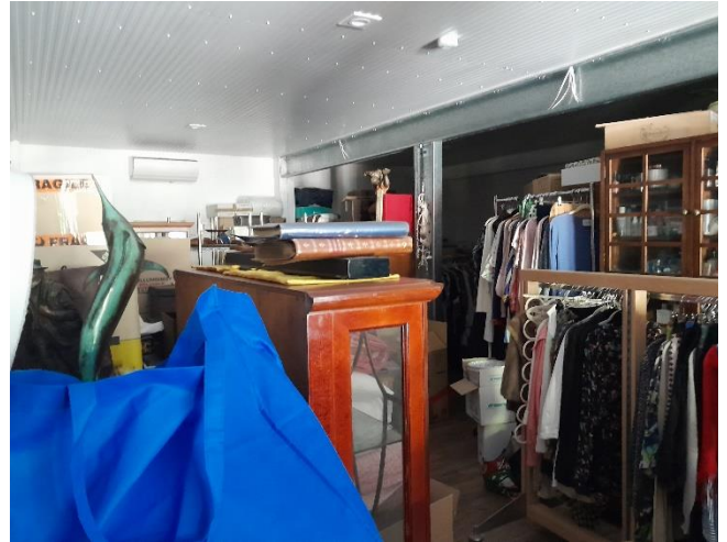
Photo 8 – Building interior – ground floor - room labelled “storage”
