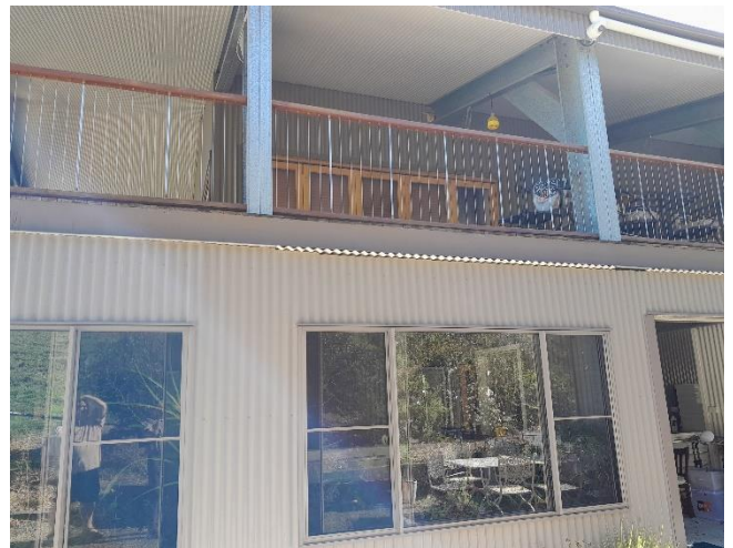
Photo 4 – Building exterior – north facade
