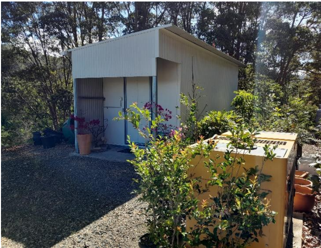
Photo 1 – Cold store – exterior
