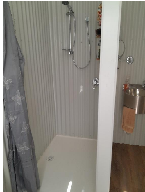
Photo 10 – Building interior – ground floor – bathroom/shower
