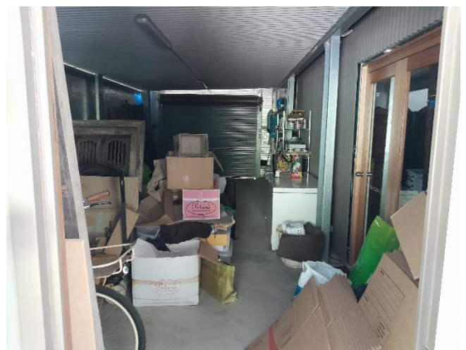
Photo 6 – Building interior – ground floor - room labelled “garage/storage”
