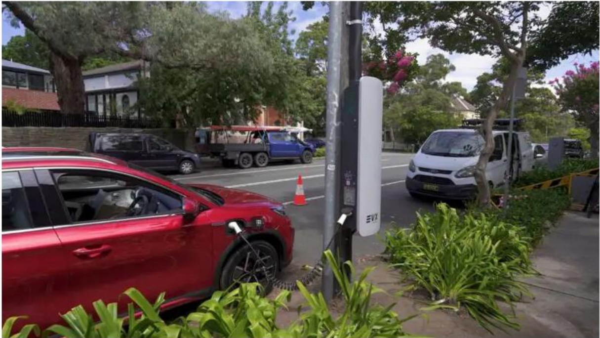
Figure 3: EVX pole mounted charger installation (Glebe, Sydney)
