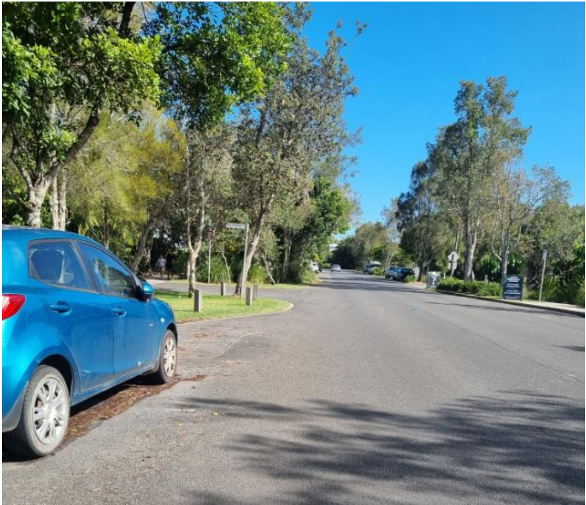
Figure 8 (above): Approach/stopping sight distance (Southbound, Bayshore Dr) at the northern intersection of Bayshore Dr/Bayshore Ln.
