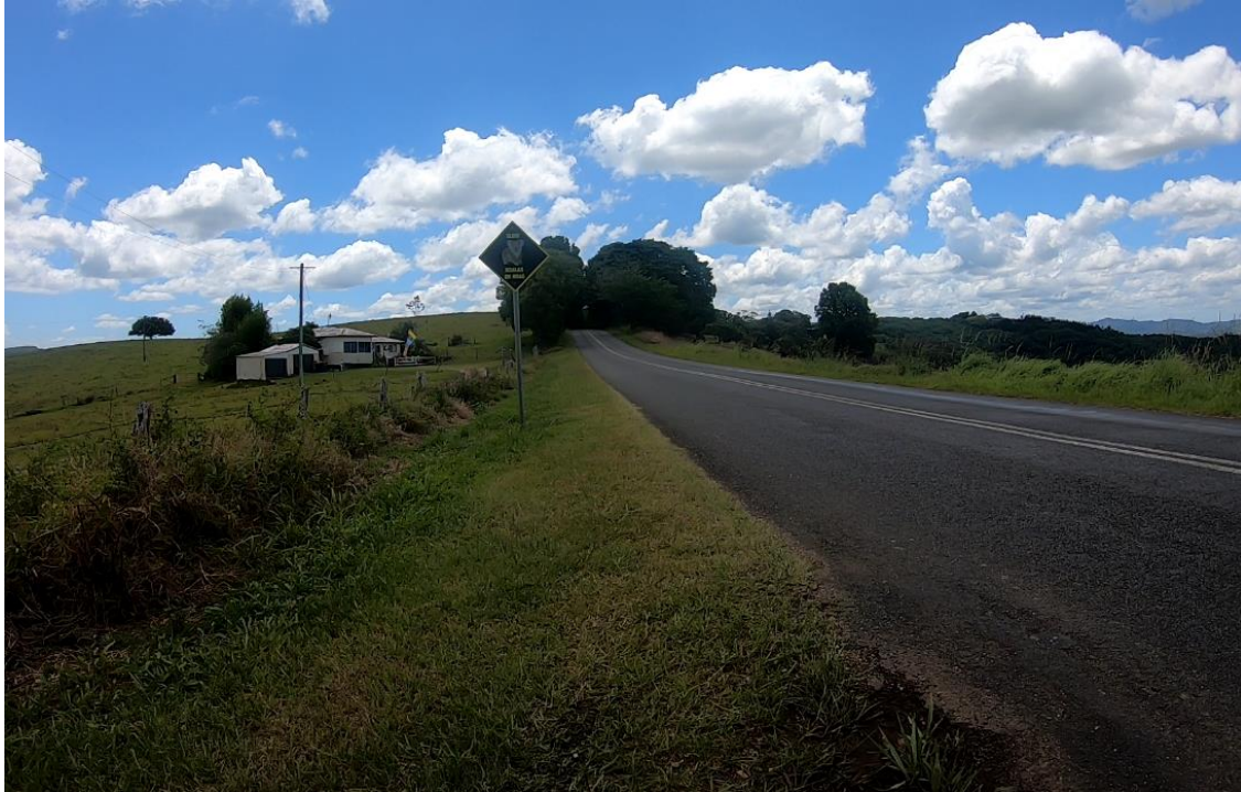
5 Figure 3: Coolamon Scenic Dr roadside environment (steep fill batter, no shoulder)
