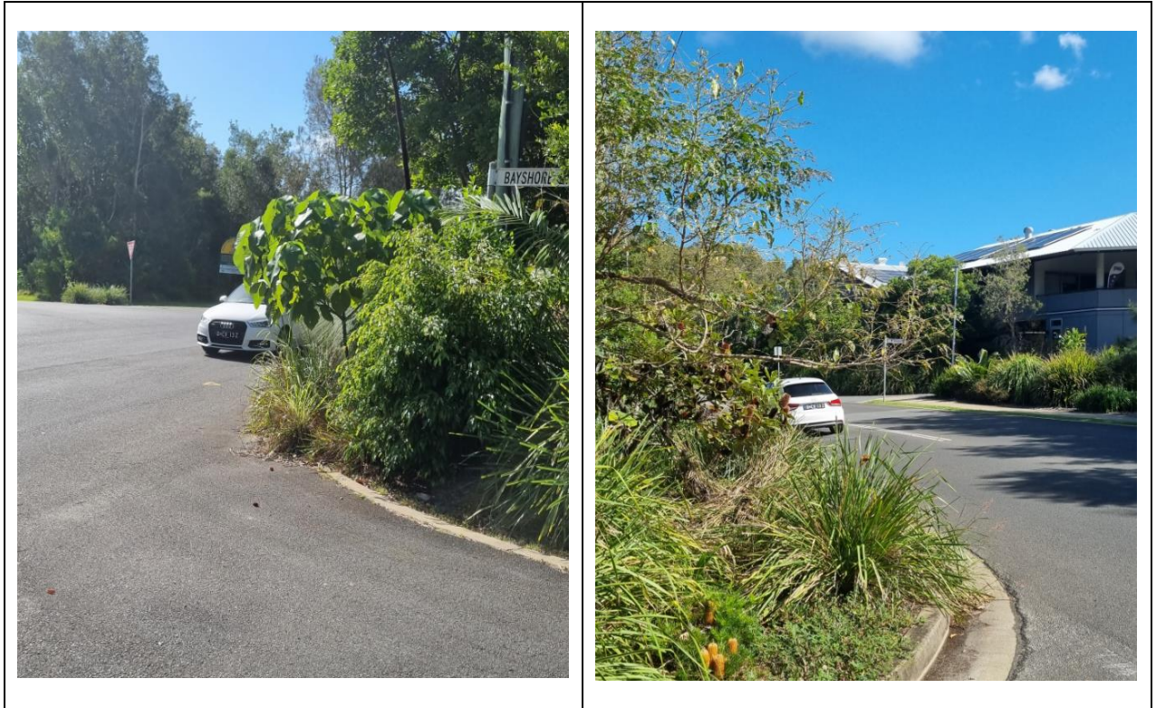
Figure 4 (above): Intersection sight distance (Bayshore Ln, South)
