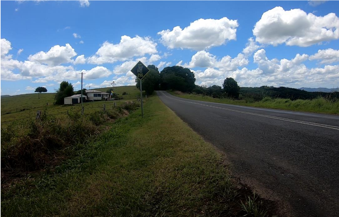
Figure 3: Coolamon Scenic Dr roadside environment (steep fill batter, no shoulder)
