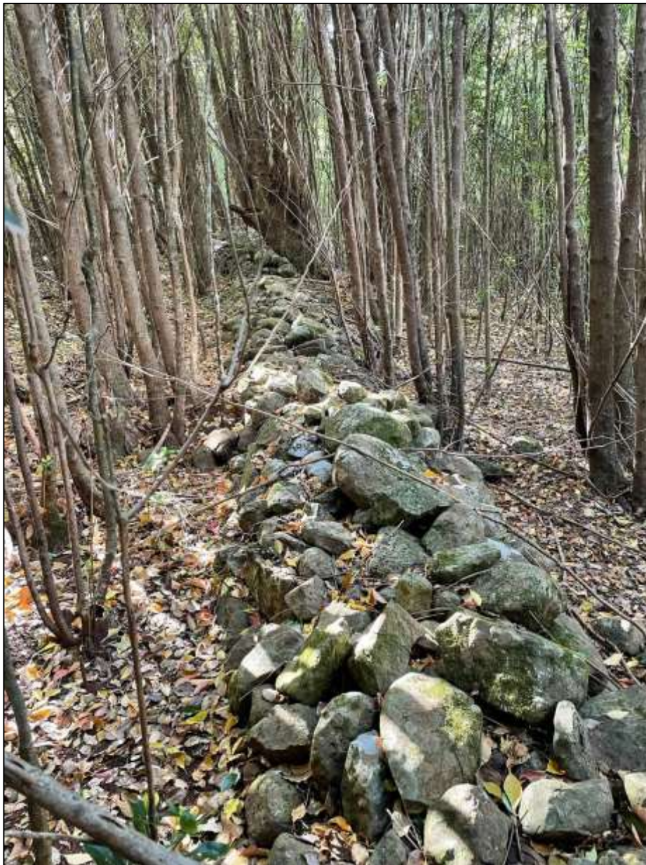
Plate 3: A constructed rock wall with potential heritage value occurs within the Vegetation Management Area. Re-shooting Camphor Laurel dominates here.
