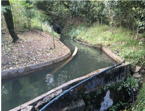
3. Water in channel and leakage from bend
