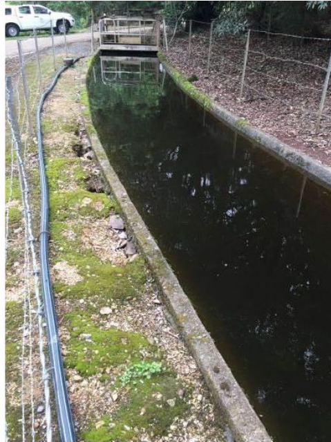
6. Sinkhole formation behind channel wall.
