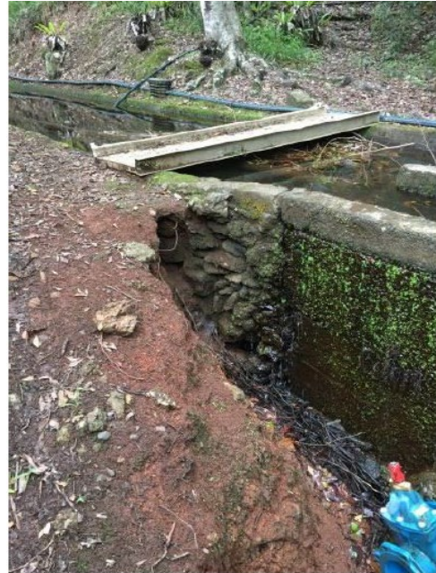
2. Scouring has removed buttressing.
