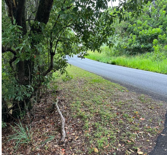
Photo 1: Sight distance left from northern driveway (Driveway A). Note vegetation obscuring sight line
