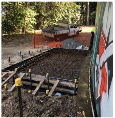
Yamble Reservoir – Access stairs slab prior to concrete pour Water Reservoir Slope Stability Works – Byron Bay and Ocean Shores
