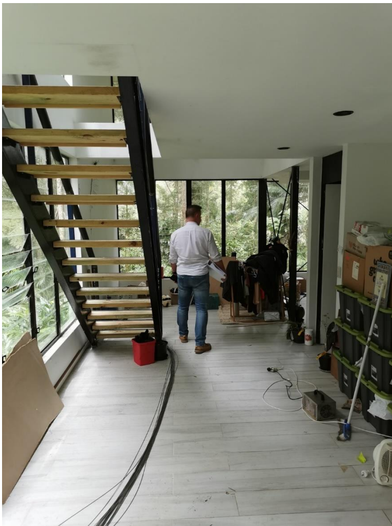
Figure 8 ground floor of structure
