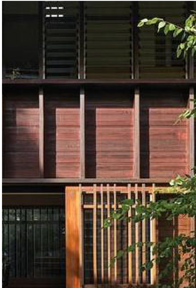
VERTICAL BATTENS & TIMBER BALUSTRADE Y3 HOUSE - DONOVAN HILL
