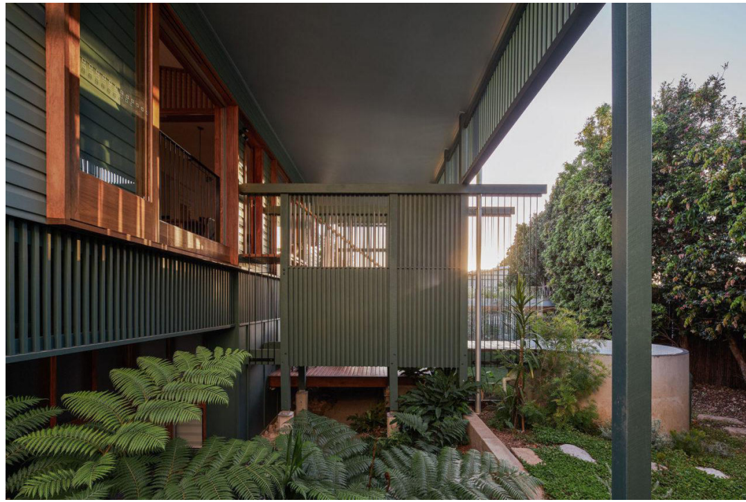
GREEN PAINTED EXTERNAL FACADE NORTHGATE ENGAWA HOUSE - ARCKE
