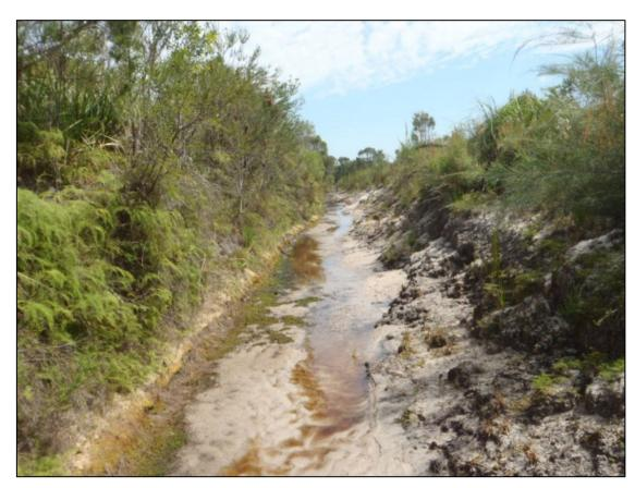
Plate 2.3 Central drain showing lack of macrophyte or sedge cover and steep partly eroded banks
