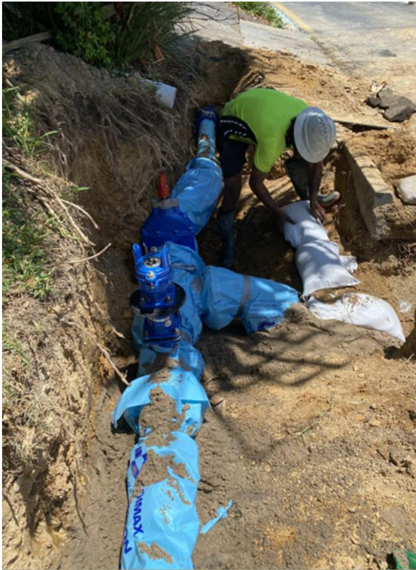
Figure 1: Site 01 Carlyle Street – Chainage 451.628 – Detail D
