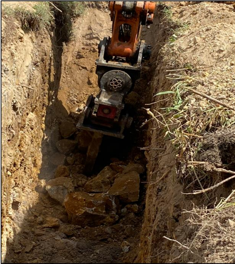
Figure 2: Site 02 Azalea St – Ch90 DN200 Trench Excavator Ripper
