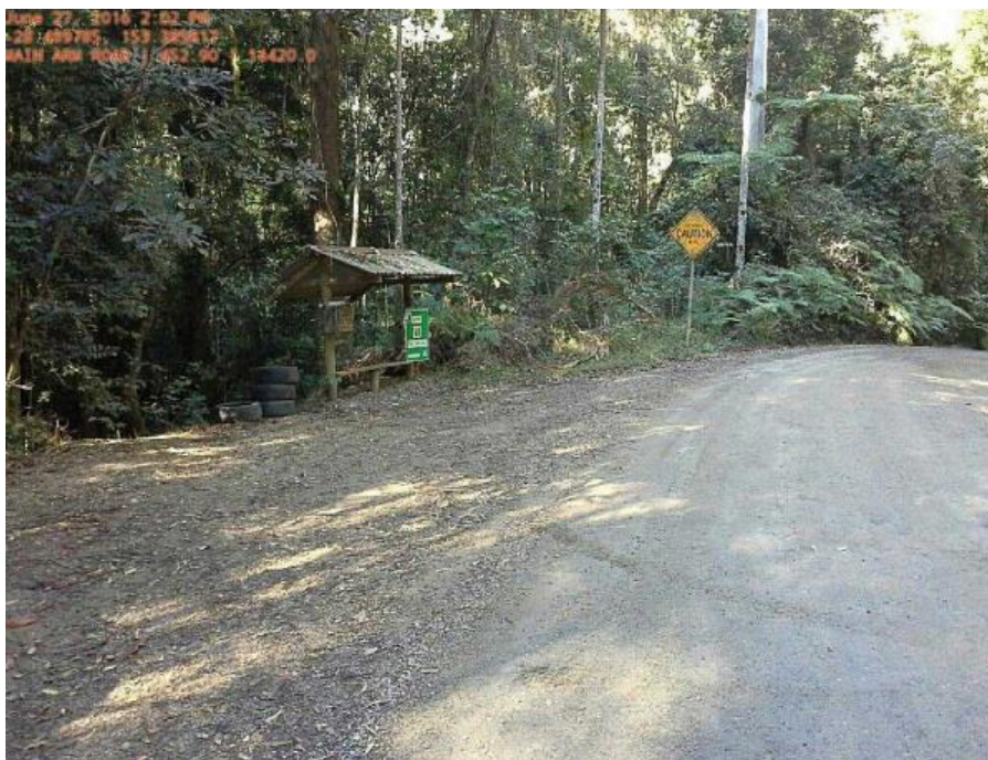
Upper Main Arm – condition 5 (very poor)
