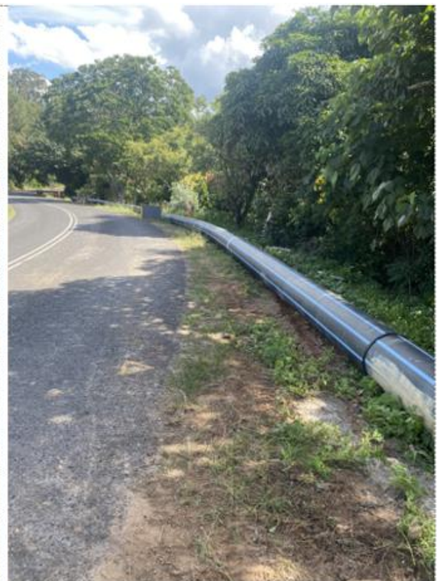
Figure 2: PE400 Pipe String Butt Welded
