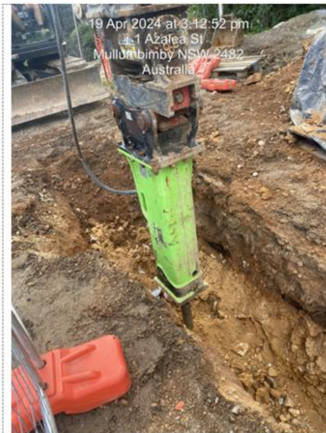
Figure 1: PE400 Trunk Main Rock Excavation
