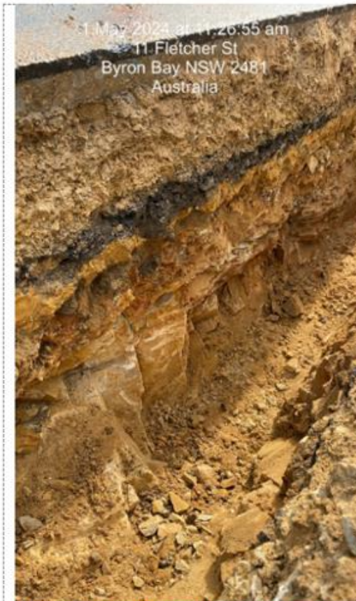
Figure 3: Fletcher St – Excavated Rock along CH60
