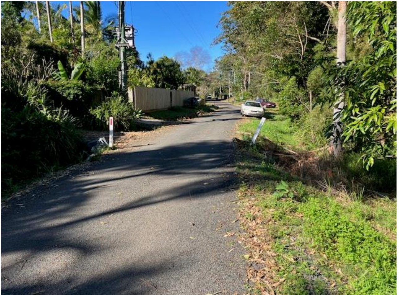
Image 7: spoon drain along the east side of road (left in photo) with culverts running under driveways and road, channelling the water to the west side of the road
