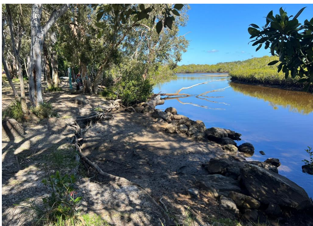
5 Figure 4: Area opposite store/café looking downstream showing ad hoc rock protection and bare riverbank
