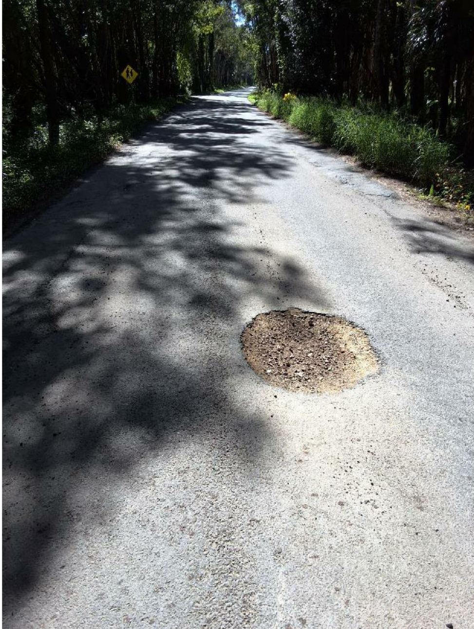
Figure 11 | Skinners Shoot Road – 5.7m seal and potholes
