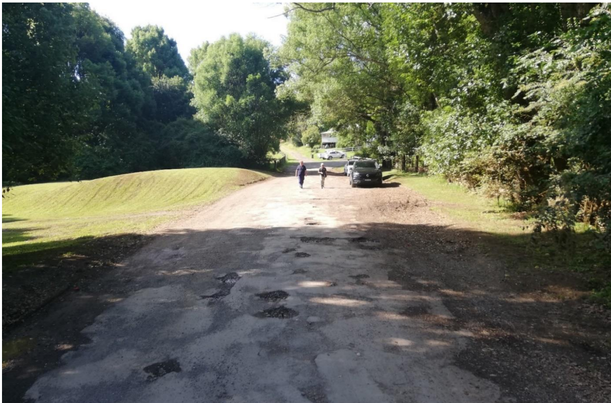
Figure 7: Entrance to the site on Cudgerie Gully Lane.
