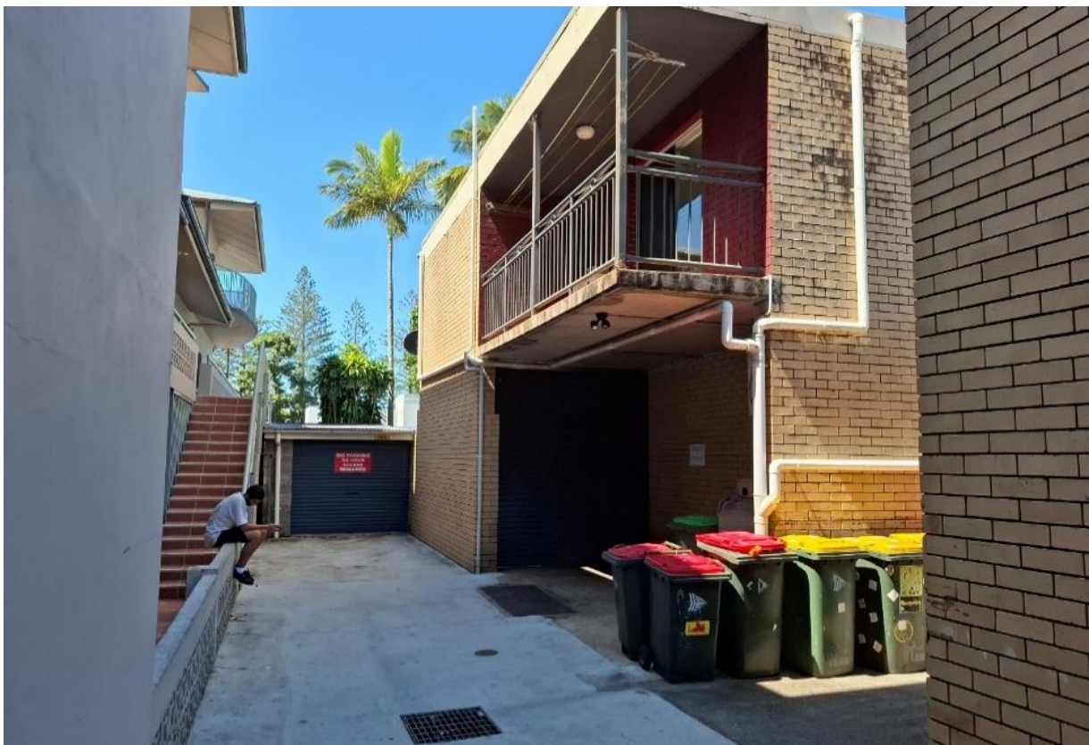
Figure 12: Rear of building.
