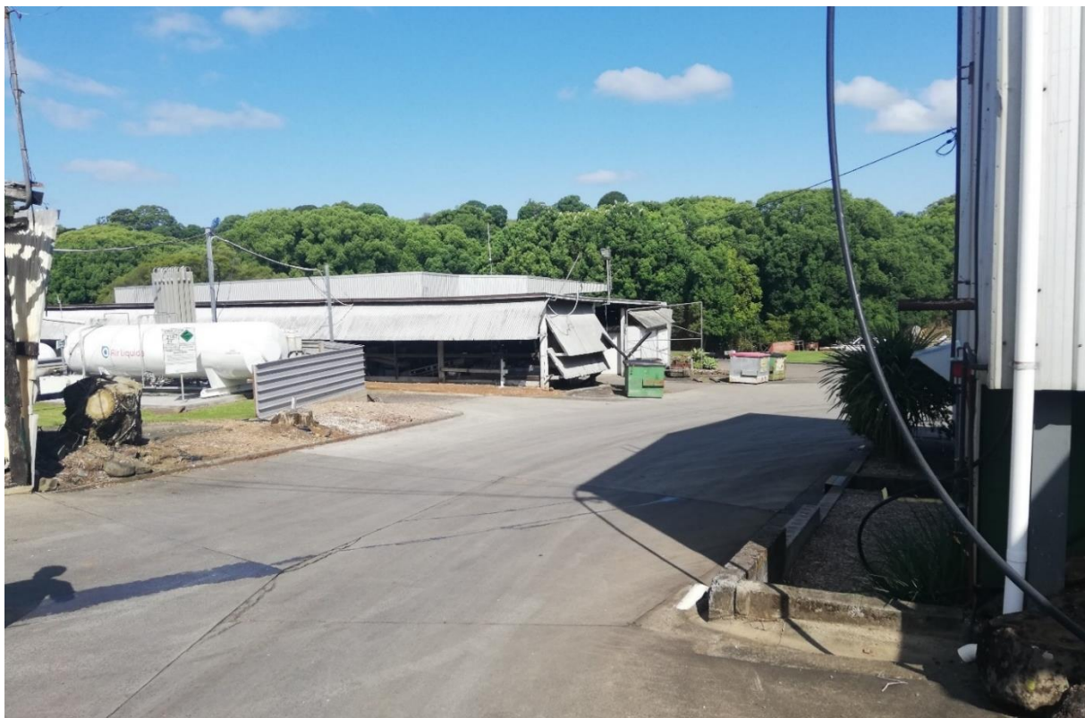
Figure 4: Main internal driveway and loading bay.
