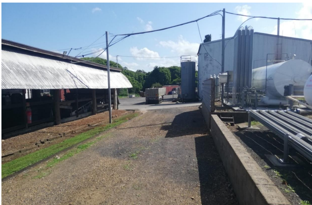
5 Figure 5: Loading bay area to be upgraded.
