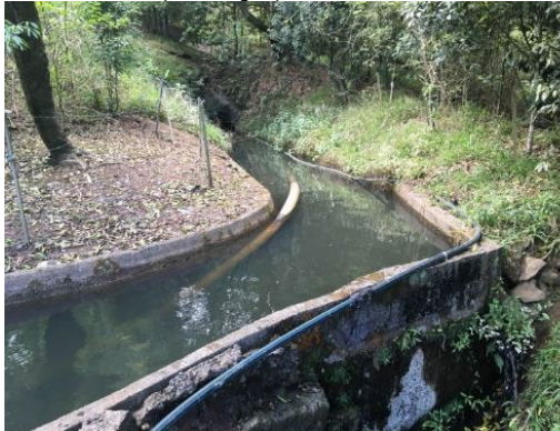
3. Water in channel and leakage from bend
