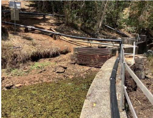
1. Channel inlet (exposed at low weir level)
