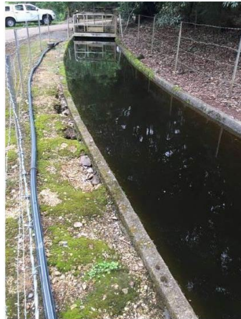
6. Sinkhole formation behind channel wall.
