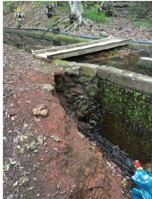
2. Scouring has removed buttressing.
