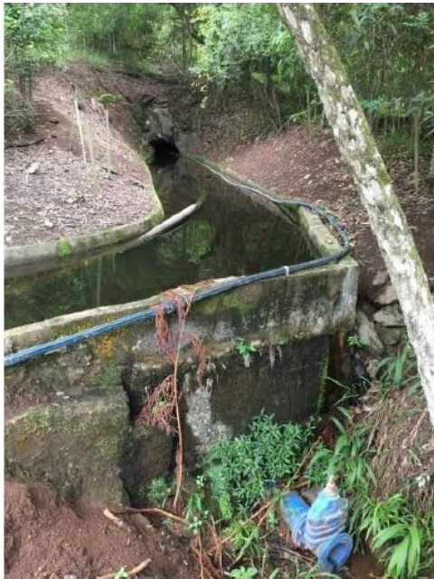
1. Subsidence and scour has exposed edges of buttress support.
