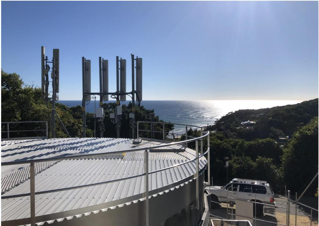
**Wategos Reservoir – Completed Roof sheeting, perimeter handrail/ kick rail, external fascia, working platforms, walkways and access hatches.**
