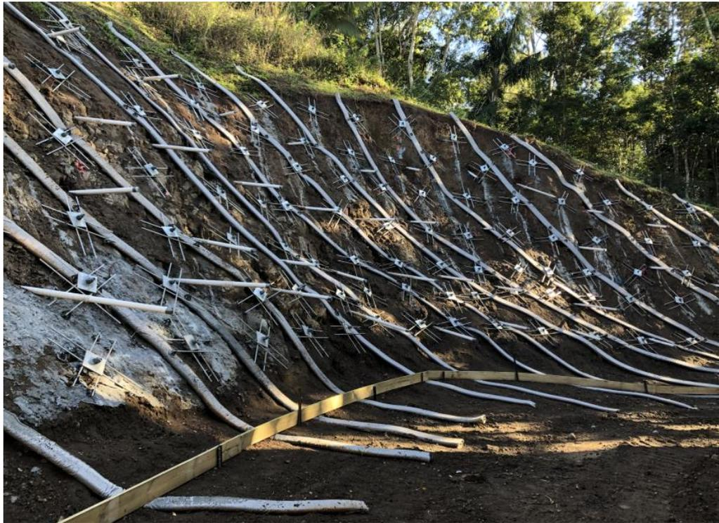
**Warrambool Reservoir – Installation of soil nails, spider plates, sub horizontal drainage, strip drains and kerb forms**
