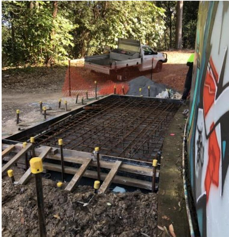
**Yamble Reservoir – Access stairs slab prior to concrete pour
