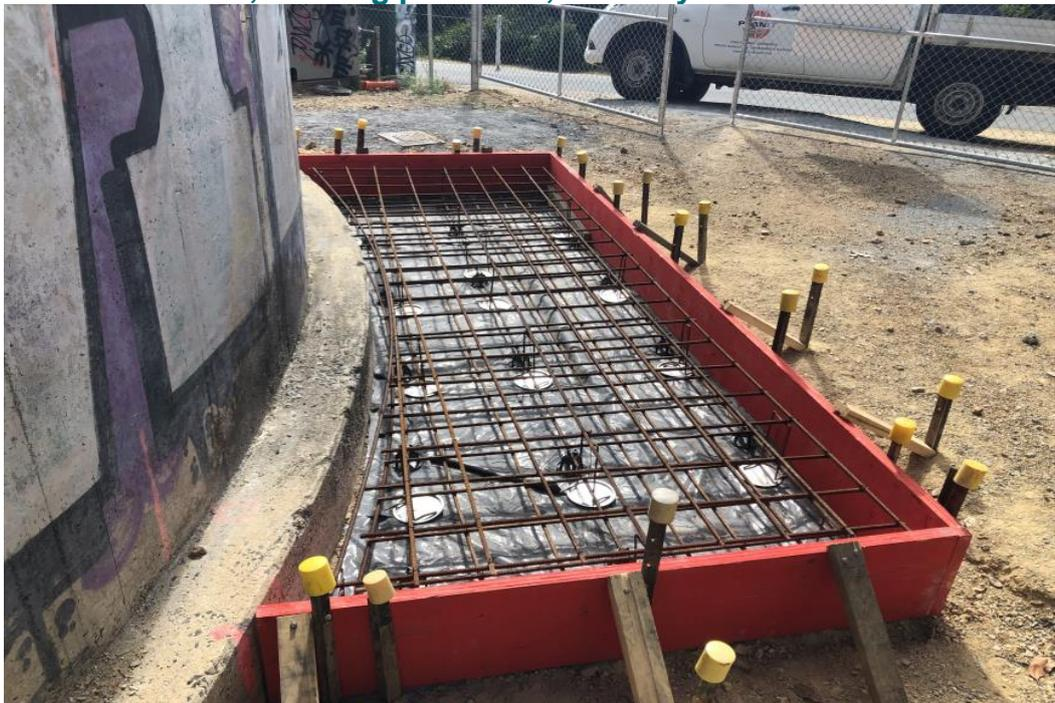
**Wategos Reservoir – Access stairs slab prior to concrete pour**
