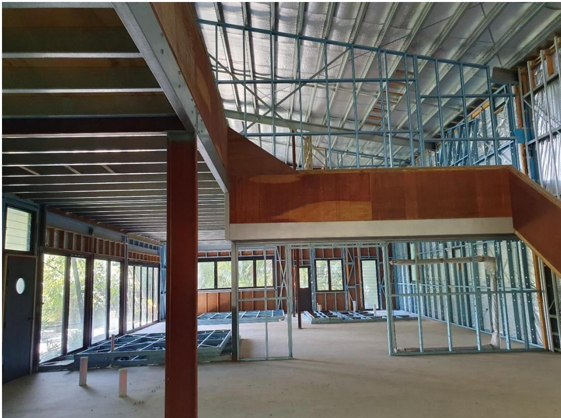
***Internal framing for dividing walls***
