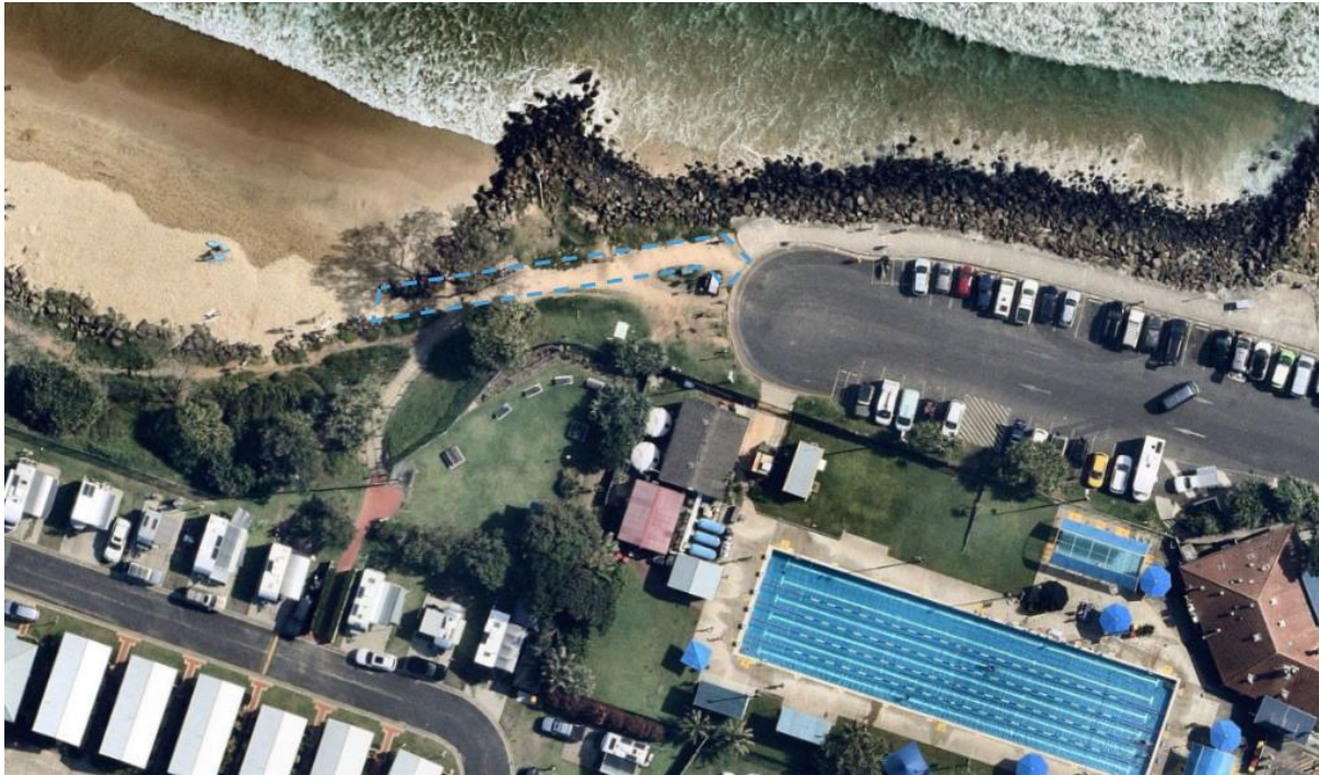
10 Figure 1: Approximate works area shown in blue dash line = western access to Belongil Beach, Byron Bay.
