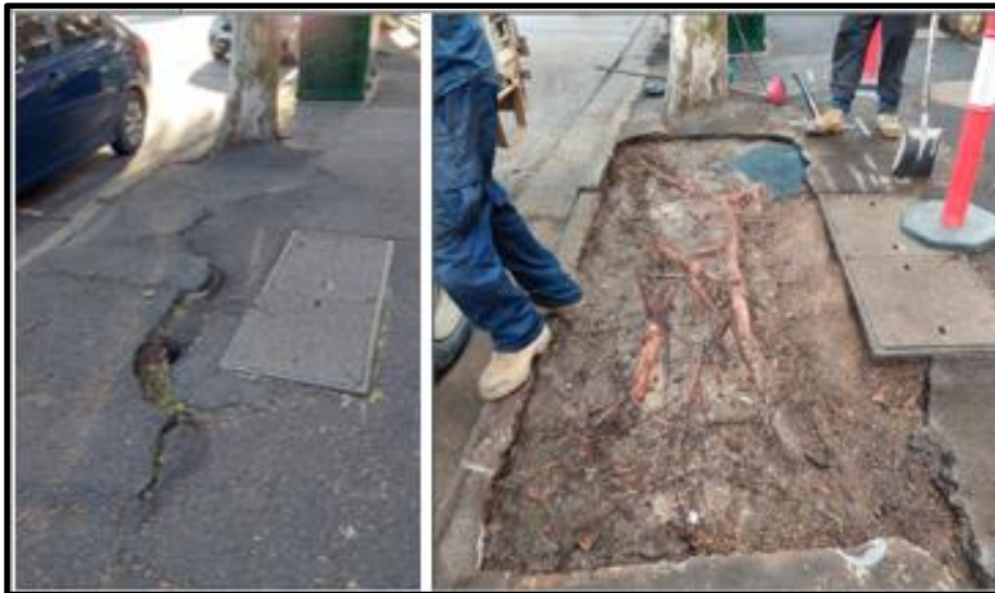
Figure 1: Leopard tree roots exposed before resealing the pavement.
