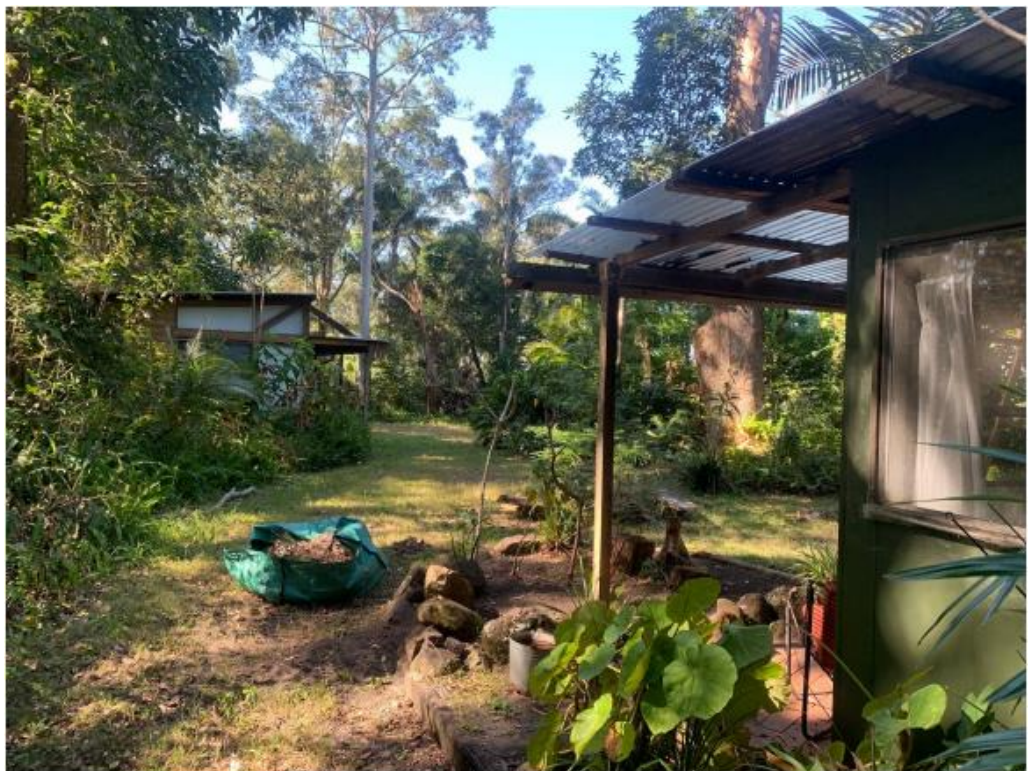
Image 3 – Building encroachments on road reserve adjoining Lot 100 DP 836091
